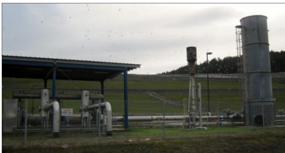
Figure 10-1: Landfill Gas Utilization Facility at Hartland Landfill
