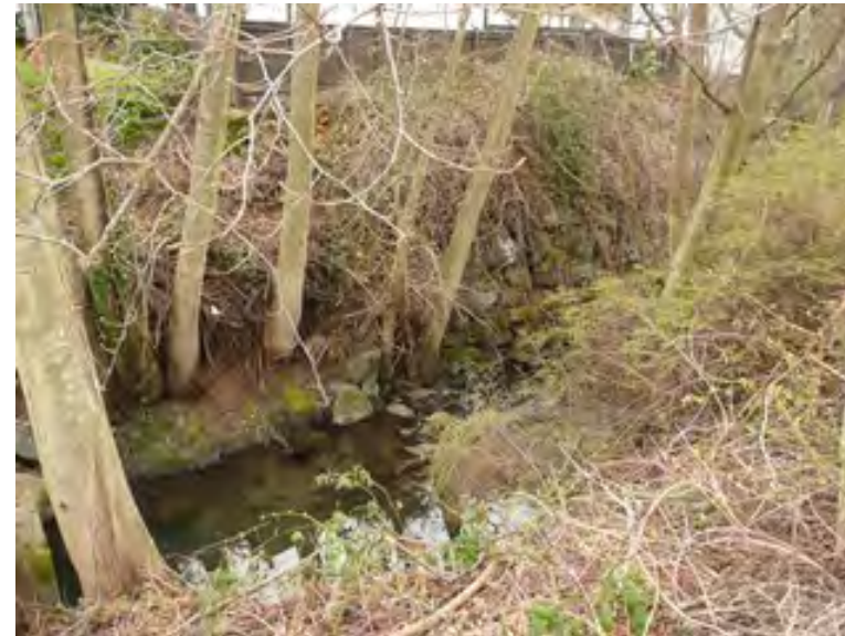
Looking across to an armoured east bank at the north end of Browning Park. The creek is highly incised at this point.
