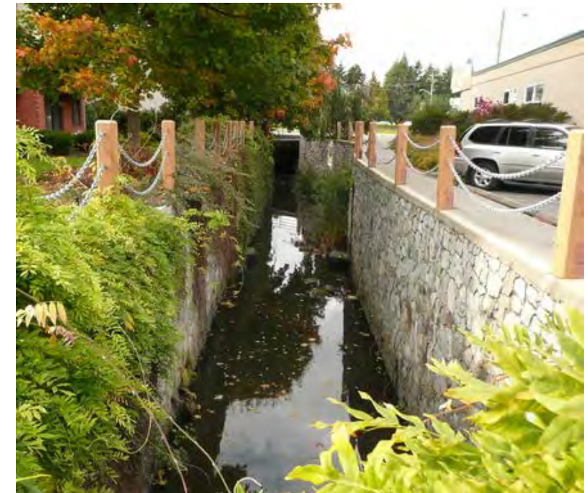
Looking upstream from Be Street. Few options exist to improve this reach. One possibility is installing in-stream baffles for complexity and aeration.
