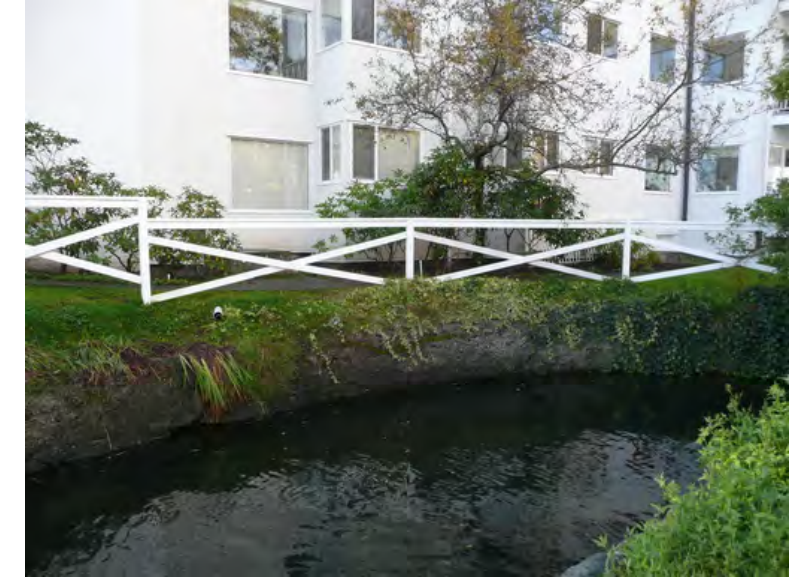
View of the rock wall showing proximity of the apartment building to the creek
