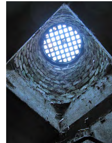
Reach 13 is entirely below ground, beneath a busy transportation corridor
