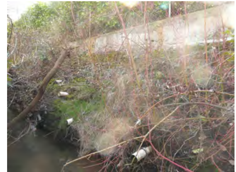
The west bank is constrained in the upper two-thirds of the reach by an extensive apartment complex at 1702 Newton Street.
