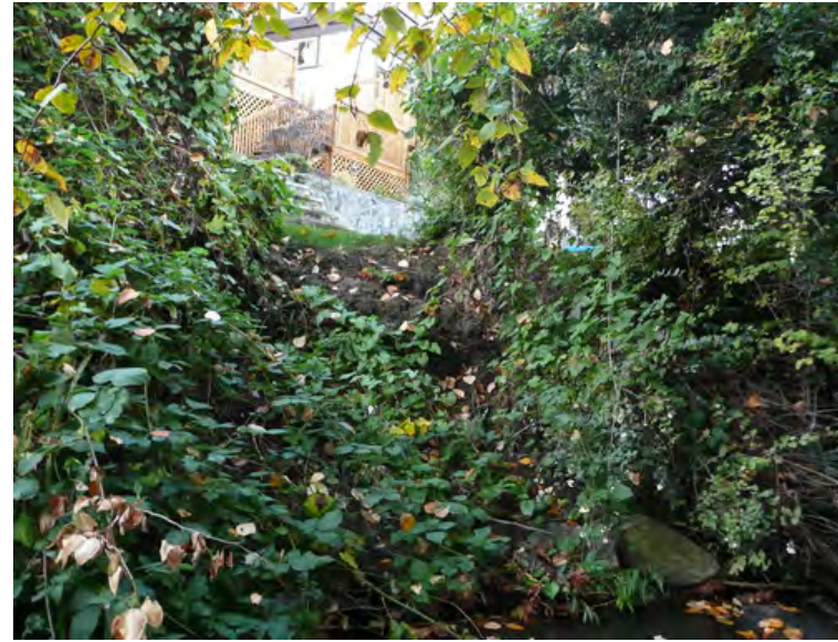
South-west corner of the Kachan property. Much of this corner has eroded away in recent years.
