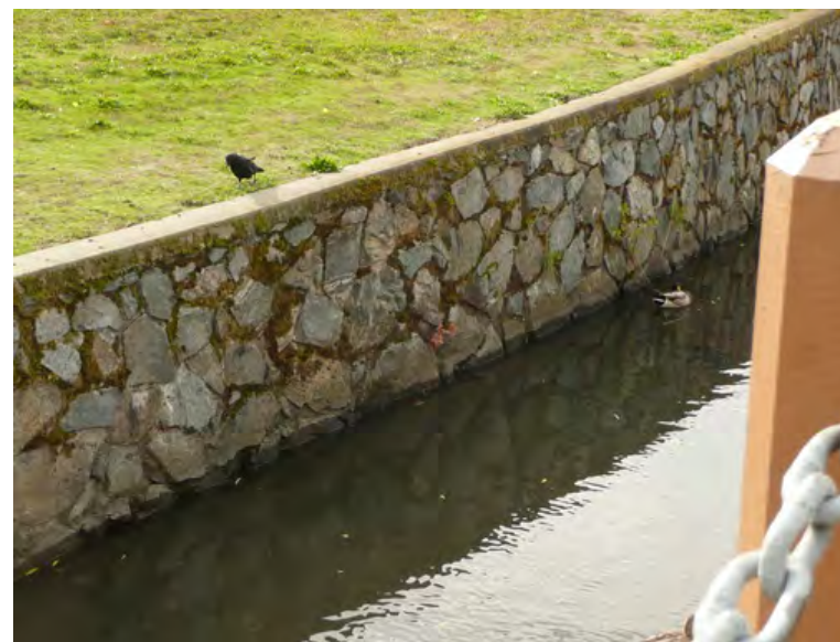
Typical concrete channel wall.
