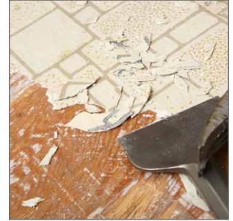
RENOVATION WASTE (residential)
