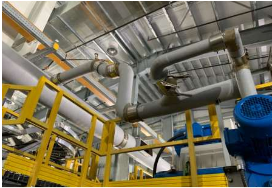
Figure 9– Residuals Treatment Facility- Installation of fibreglass ducting for odour control system ongoing in Residuals Handling Building.
