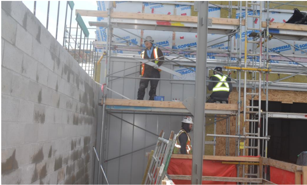
Figure 3– McLoughlin Point Wastewater Treatment Plant- Cladding installation on north end of heat recovery room.
