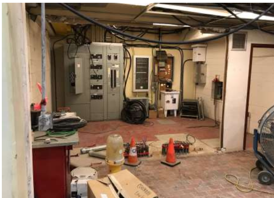
Figure 11–Clover Point Pump Station- Electrical equipment demolition in the old electrical room.
