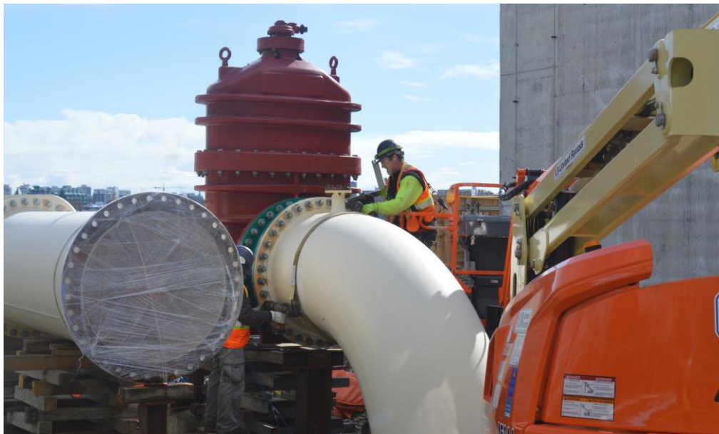
Figure 2– McLoughlin Point Wastewater Treatment Plant - Bolting up valve and fittings at pigging chamber preparing for pressure test.
