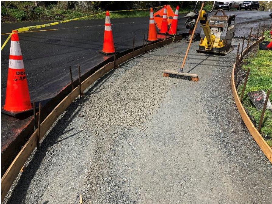
Figure 23–Residual Solids Pipes - Sidewalk, curb and gutter preparation on corner of Burnside Road and Grange Road.
