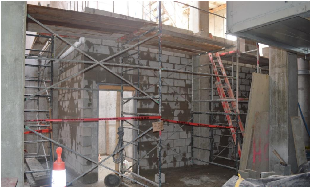
Figure 6– McLoughlin Point Wastewater Treatment Plant- Cinder block installation at northeast stairwell of tertiary treatment structure.
