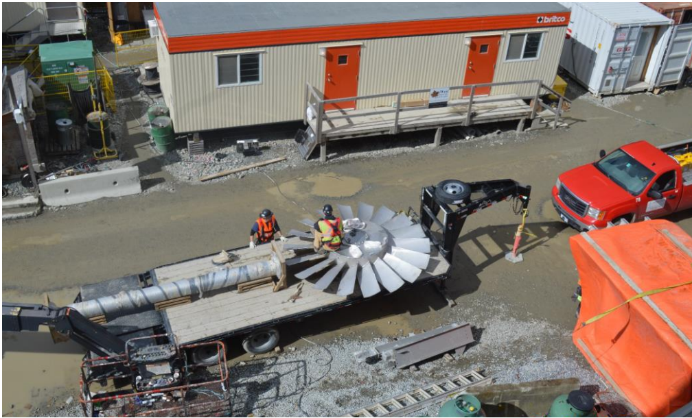
Figure 5– McLoughlin Point Wastewater Treatment Plant- delivery of turbine blade for Densadeg reactor.
