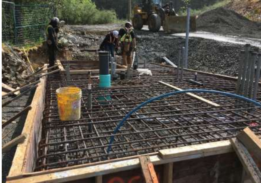
Figure 23 –Residual Solids Pump Stations – Pump Station 3 Installing formwork and rebar for odour control unit slab.
