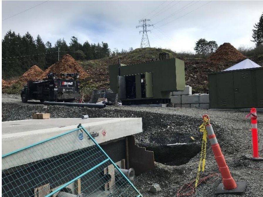
Figure 24–Residual Solids Pump Stations– Pump Station 3 – Emery Electric performing a 5– hour load test on the generator.
