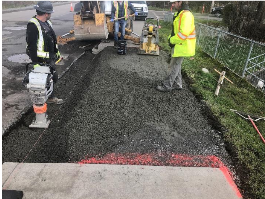
Figure 20– Residual Solids Pipes-Sidewalk, curb and gutter preparation on Interurban Road at Charlton Road
