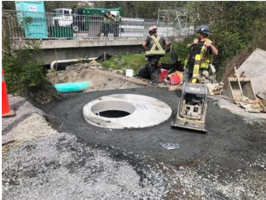
Figure 18- Residual Solids Pipes- Backfill and compaction around line valve at Admirals Bridge.
