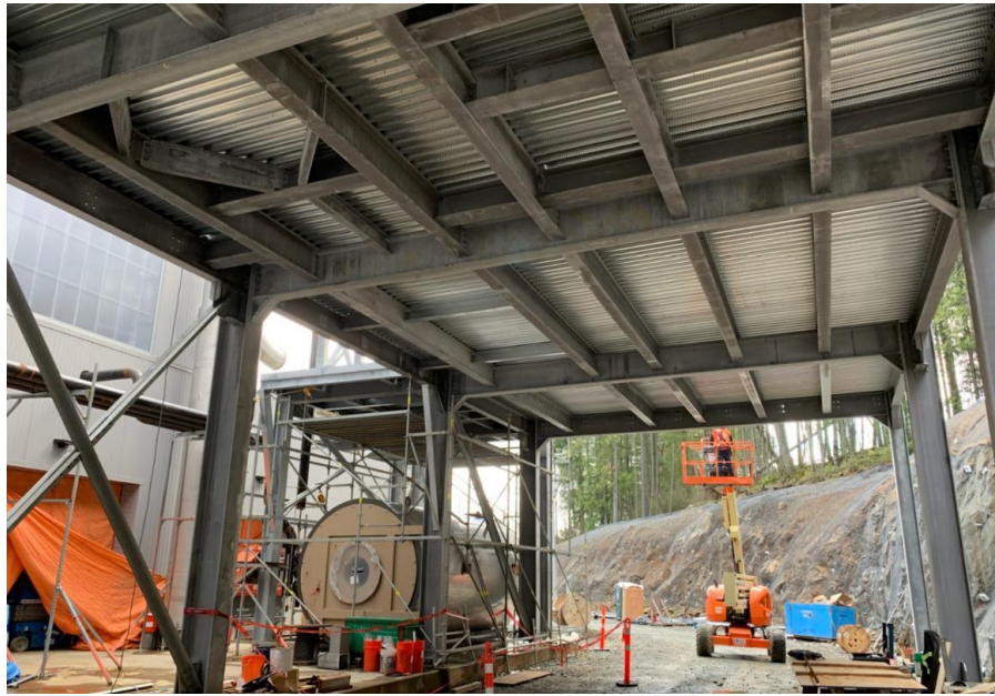
Figure 8– Residuals Treatment Facility- Installation of Q deck roofing system ongoing on product load out structure.
