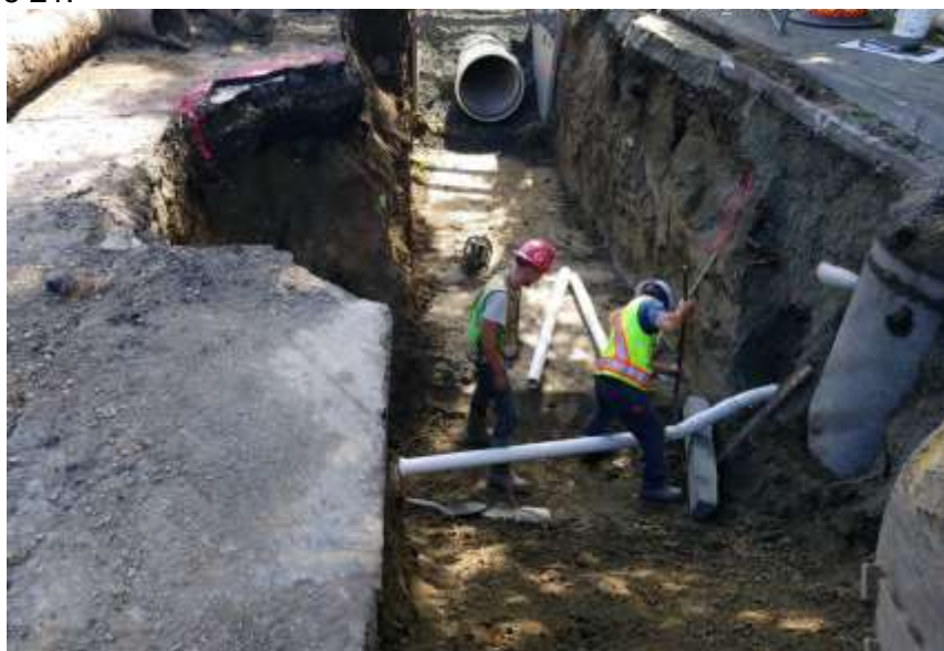
Figure 21- Trent Forcemain – Stannard Avenue – Realignment of sanitary service at Fairfield Road.
