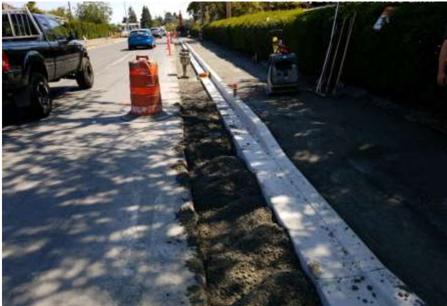
Figure 21–Trent Forcemain- Fairfield Road curb and sidewalk subgrade preparation.
