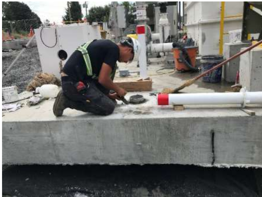
Figure 17–Residual Solids Pump Stations– Pump Station 1 –Installing bollard sleeves on the Odour Control pad.
