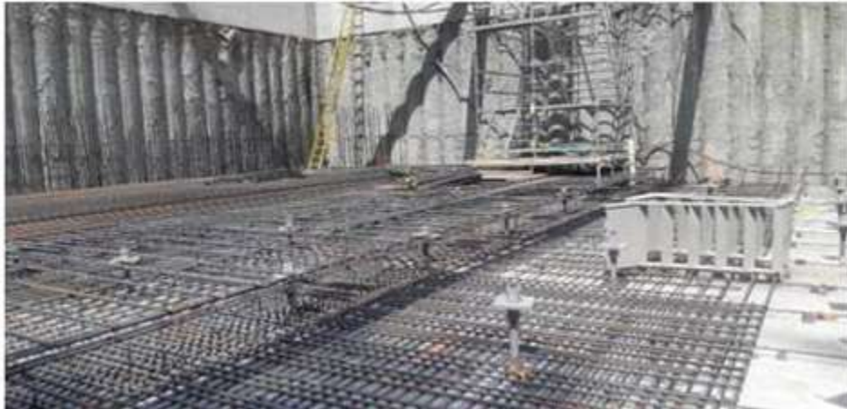
Figure 19–Arbutus Attenuation Tank- Base Slab Steel Installation Progress.
