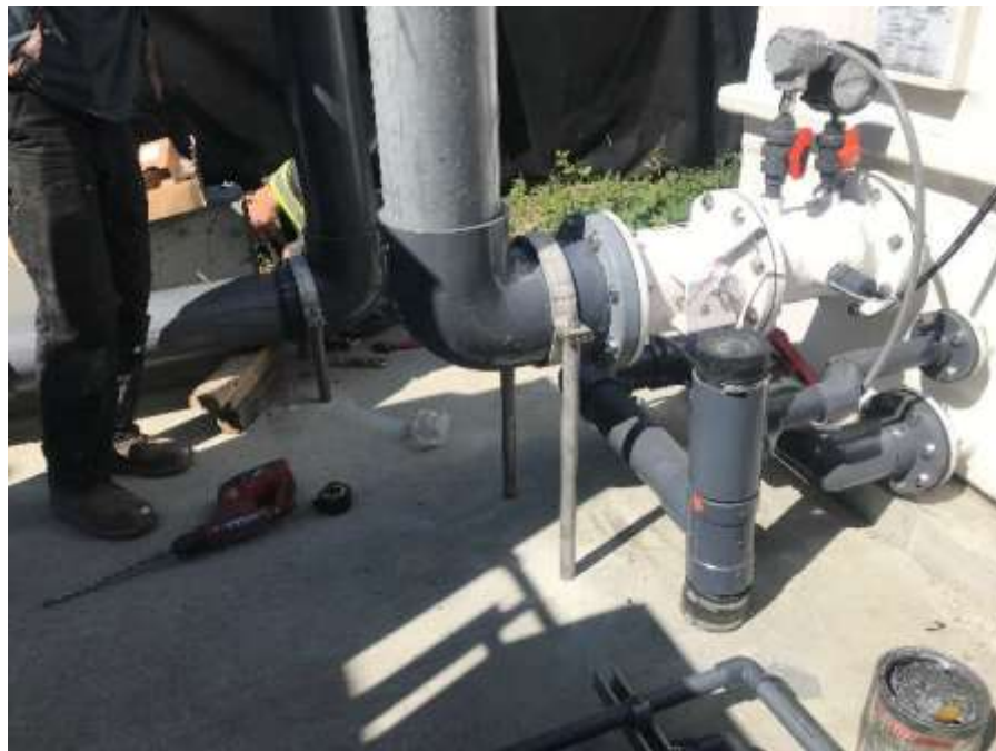
Figure 19 –Residual Solids Pump Stations – Pump Station # 1: installing pipe stands on the Odour Control Unit vent piping.
