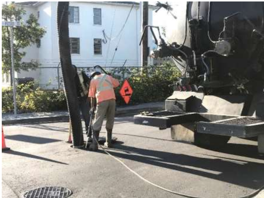
Figure 15- Residual Solids Pipes- Pressure washing manhole at Lyall Street and Peters Street.
