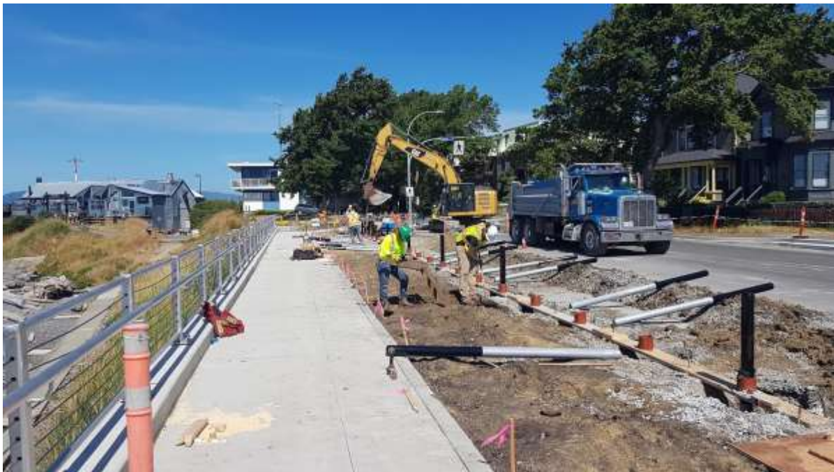
Figure 13–Clover Forcemain- Installing parking bollards along Dallas Road
