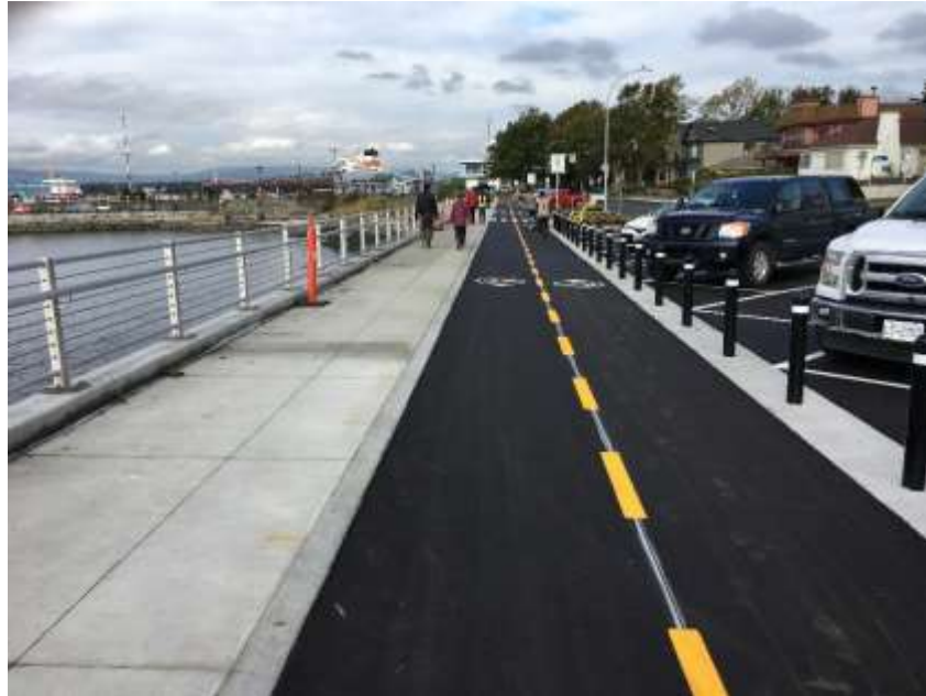
Figure 13–Clover Forcemain- Cycle track with lines painted, bollards installed and sidewalk and fence complete.
