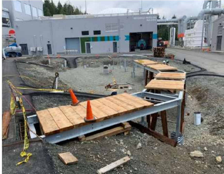
Figure 6– Residuals Treatment Facility- Construction of boardwalk in storm pond north of operations building.
