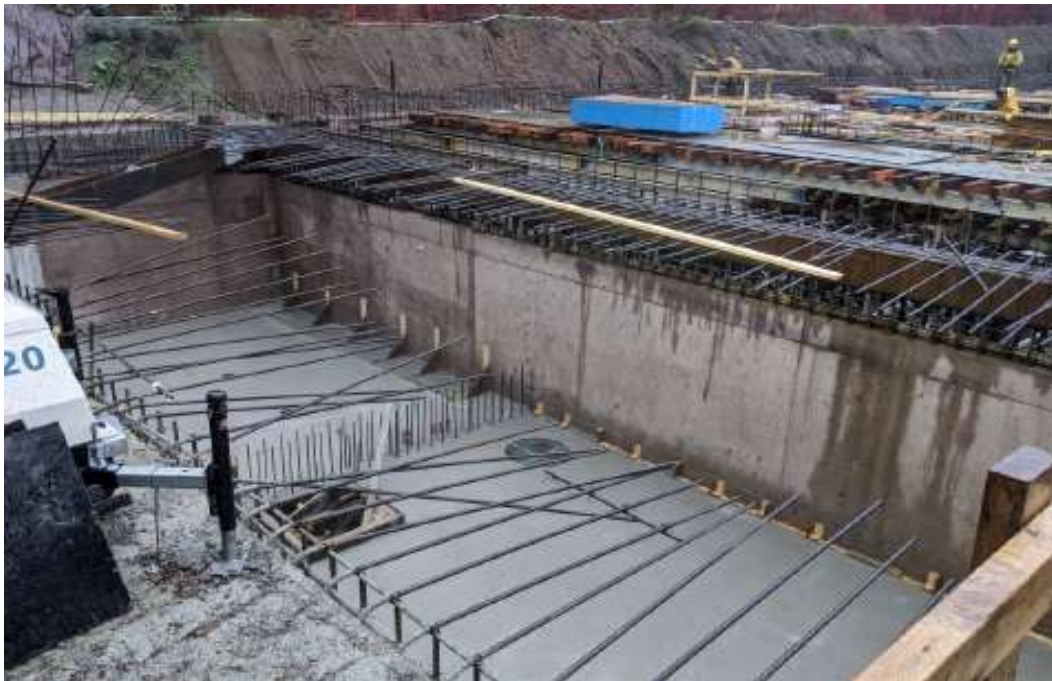
Figure 14–Arbutus Attenuation Tank- Concrete Pour completed at the South end of the tank
