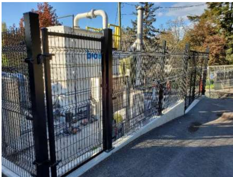
Figure 18–Residual Solids Pump Stations–Pump Station 2 – Single and double gates for the Omega fence around the odour control unit were installed
