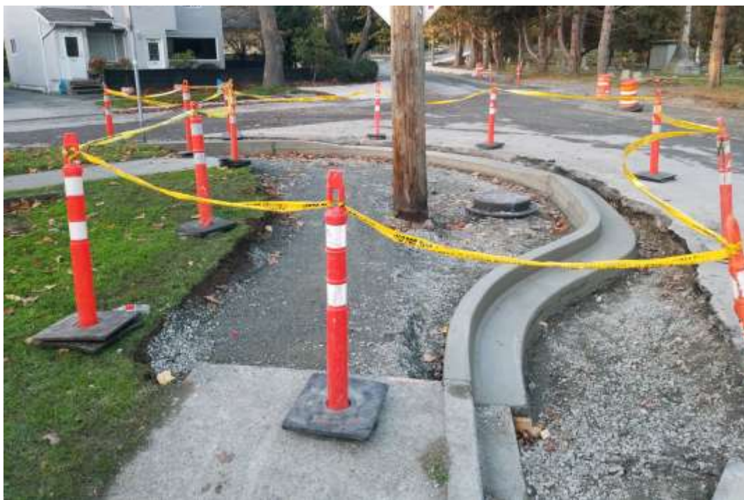
Figure 22–Trent Forcemain- Poured curbing at the intersection of Memorial Crescent and Bushby Street.
