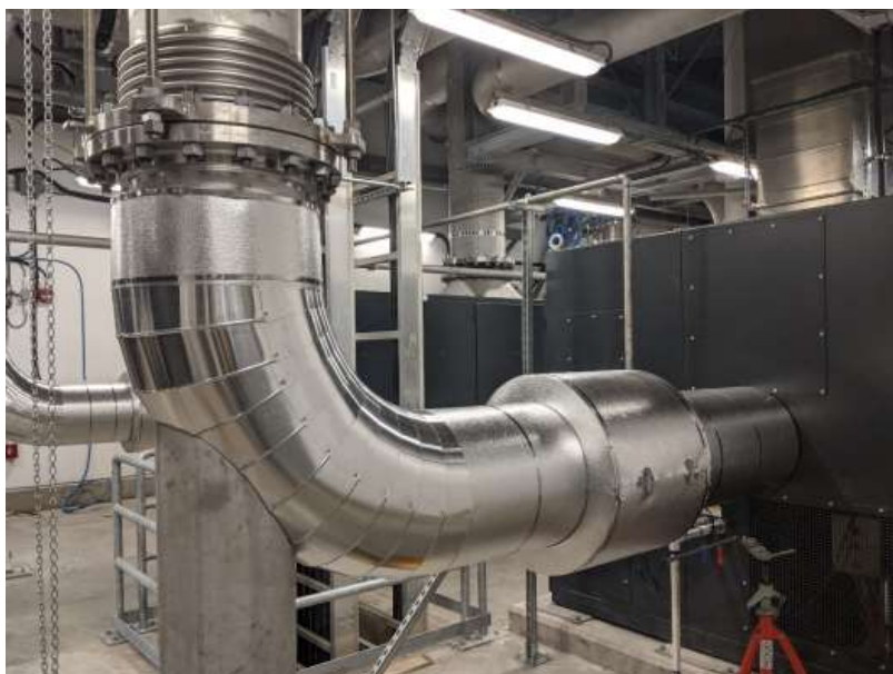
Figure 2– McLoughlin Point Wastewater Treatment Plant- Blower outlet process air piping insulation installed.
