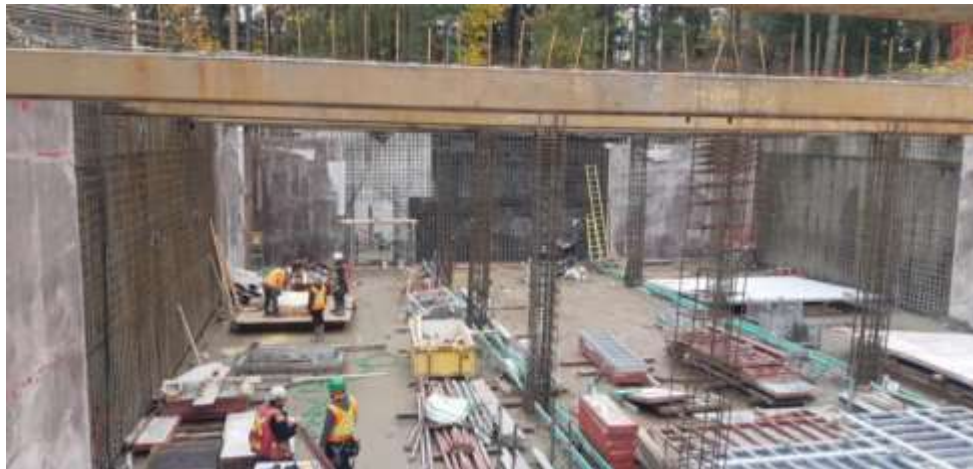
Figure 12 – Arbutus Attenuation Tank- Column reinforcing installation process.
