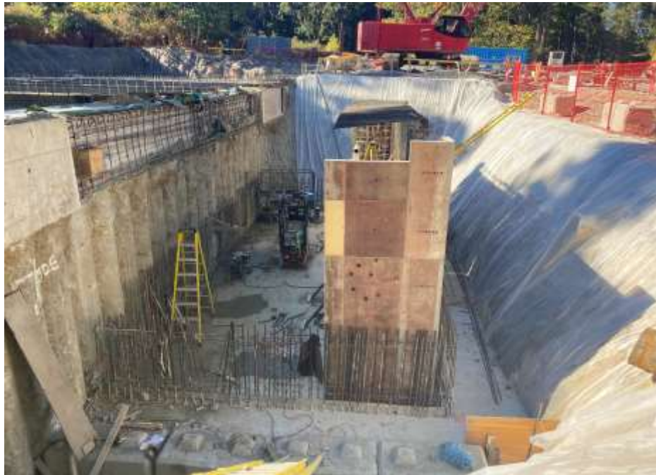
Figure 18–Arbutus Attenuation Tank- Valve chamber wall formwork installed.
