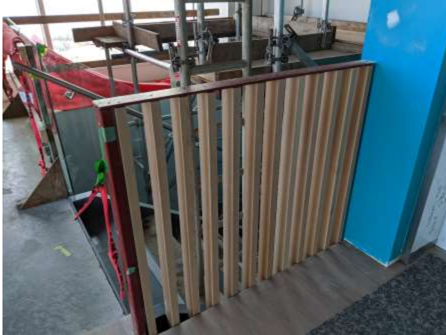
Figure 2– McLoughlin Point Wastewater Treatment Plant – Railing installation in Operations & Maintenance building main entrance stairway.
