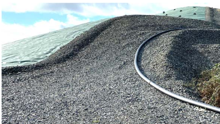
Photos 4.8a & 4.8d - Emission Hotspots, Edge of Geomembrane Liner and Damaged Liner (Area S1)
