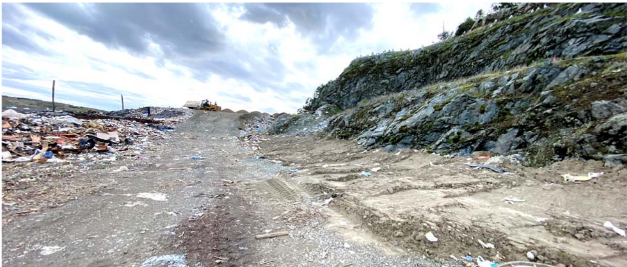
Photo 4.5 - Rock Wall Drainage Blanket Clay Plug, October 2020
