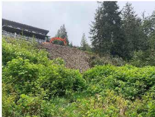
Photo 4. View looking south at the excavated soil being placed along the northern development boundary outside of the 15m Shoreline Protection DPA. May 14, 2021.
