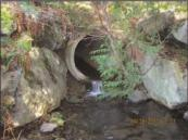
Photo 7 Seedtree Road concrete culvert conveying Seedtree Creek (C. Barlow).
