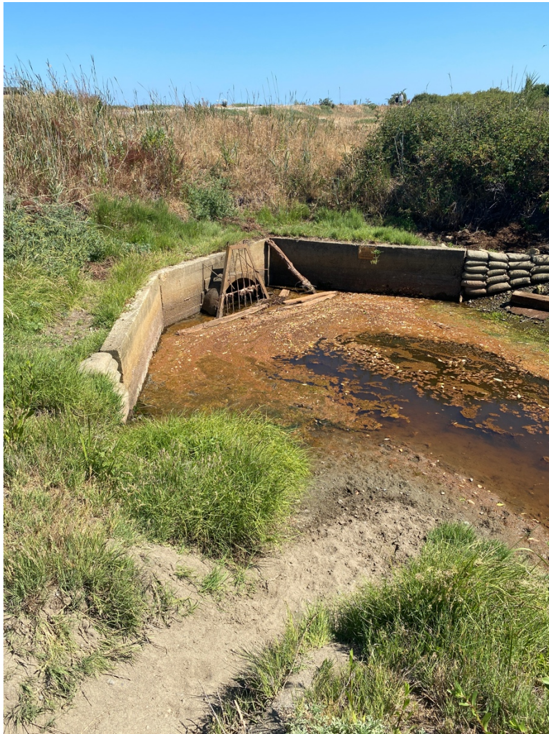
Figure 46. Trash rack upstream of tide gate. July 5, 2021.
