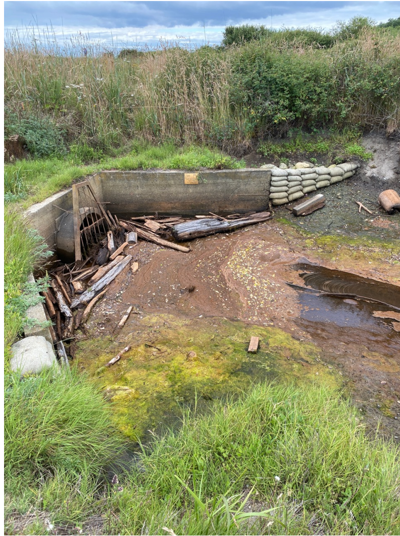
Figure 47. Trash rack upstream of tide gate. July 7, 2020.
