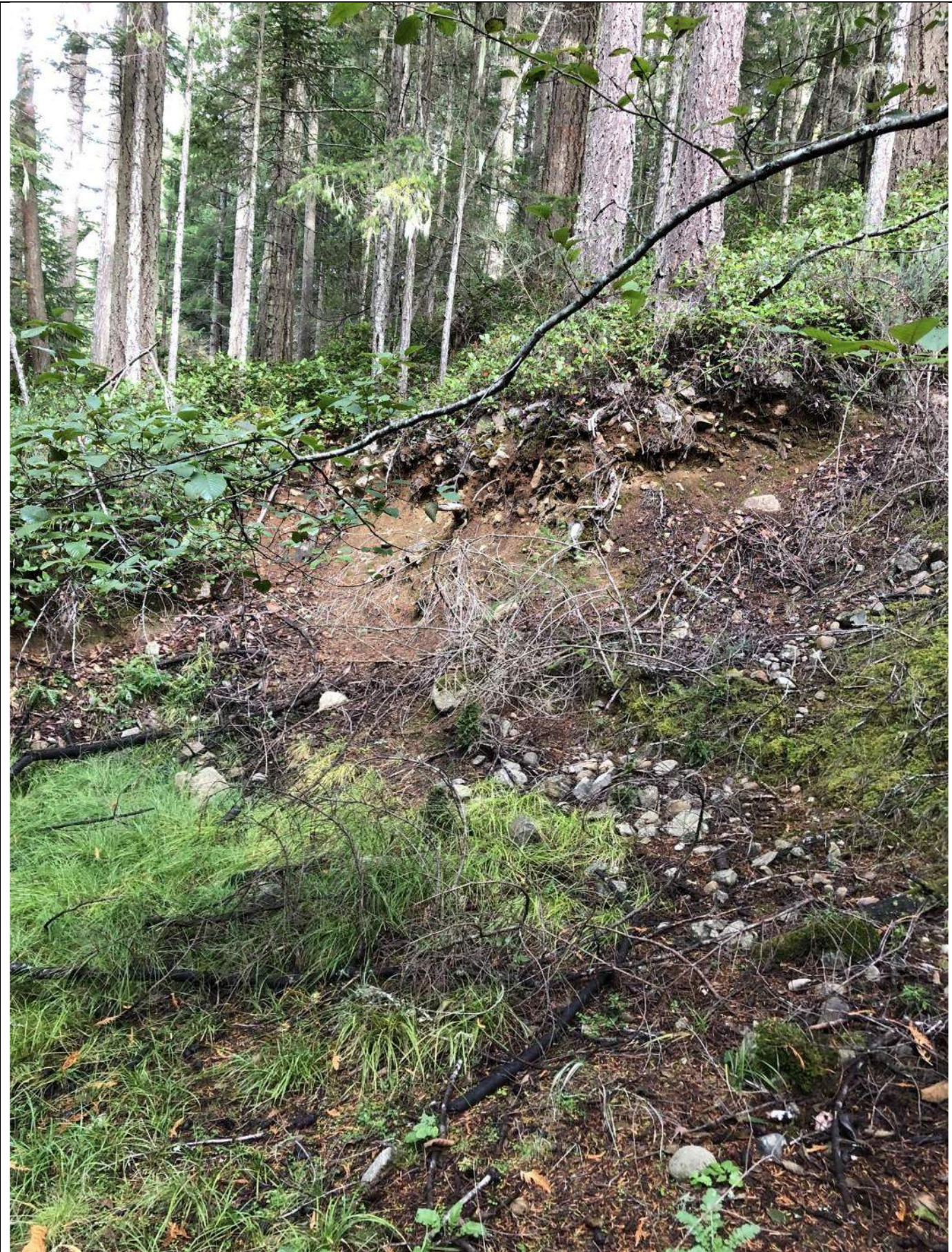
Photo 01: Sloughing and slope erosion near basin associated with ephemeral stream east of reservoir.
