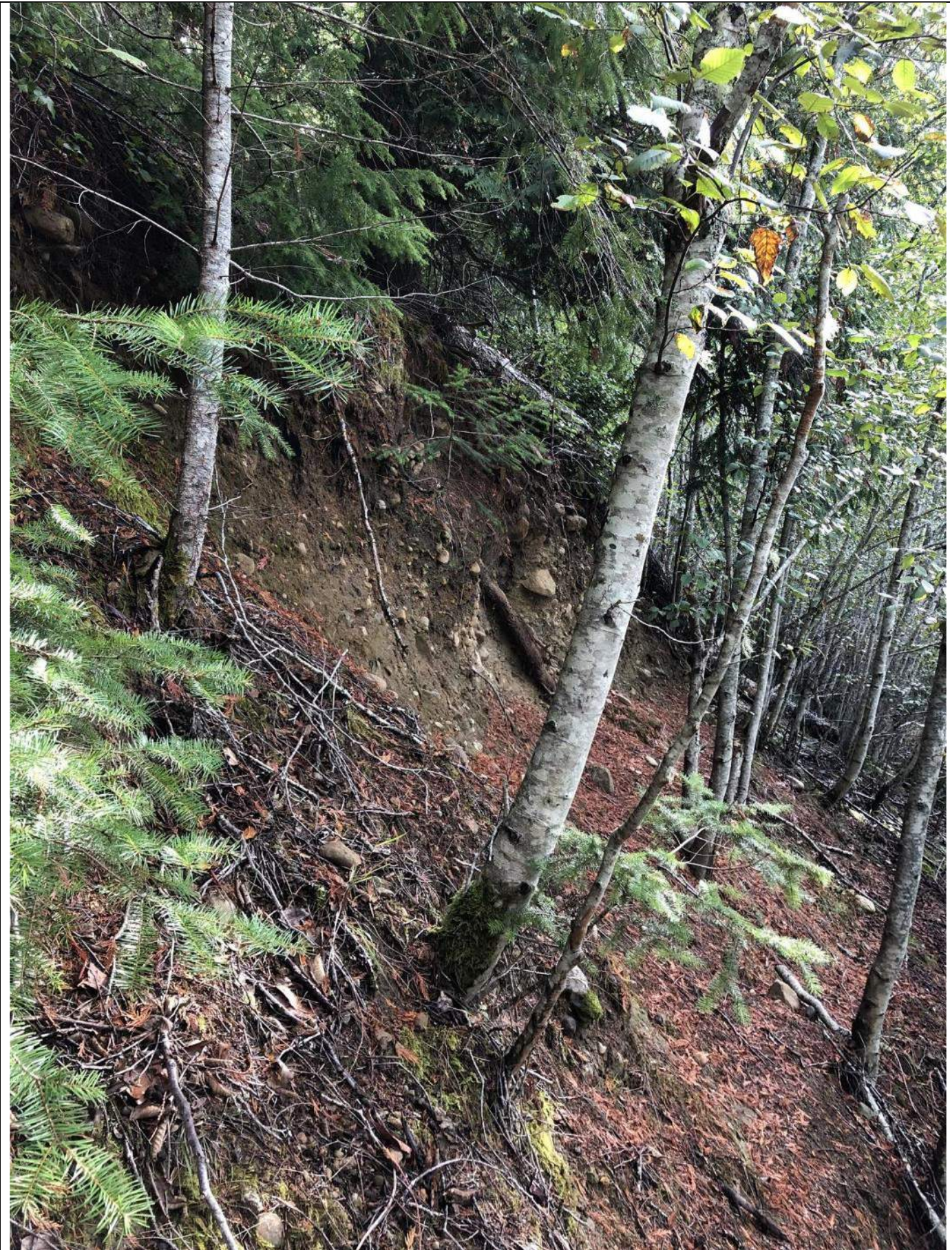
Photo 08: Sloughing/slope erosion observed just above the eastern waterline of the reservoir (Photo 2 of 2).
