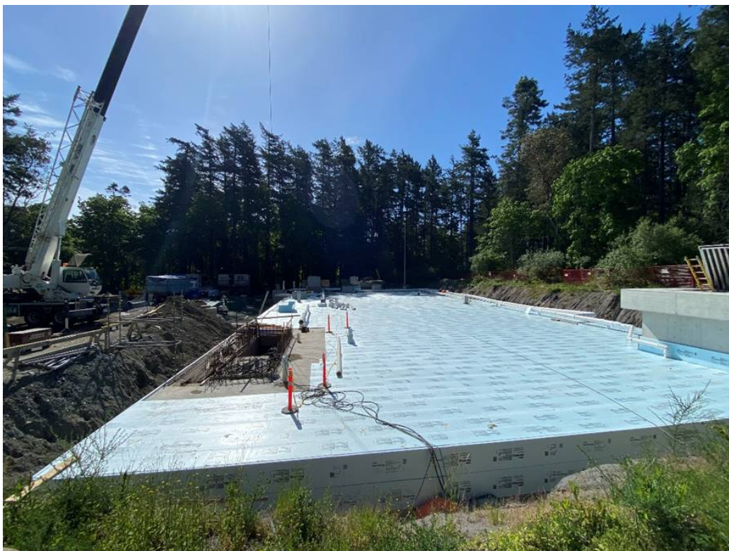
Figure 14 – Arbutus Attenuation Tank (Construction in progress)
