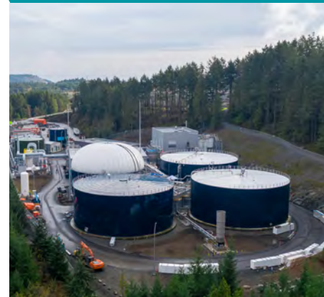
Residuals Treatment Facility, Victoria, BC
