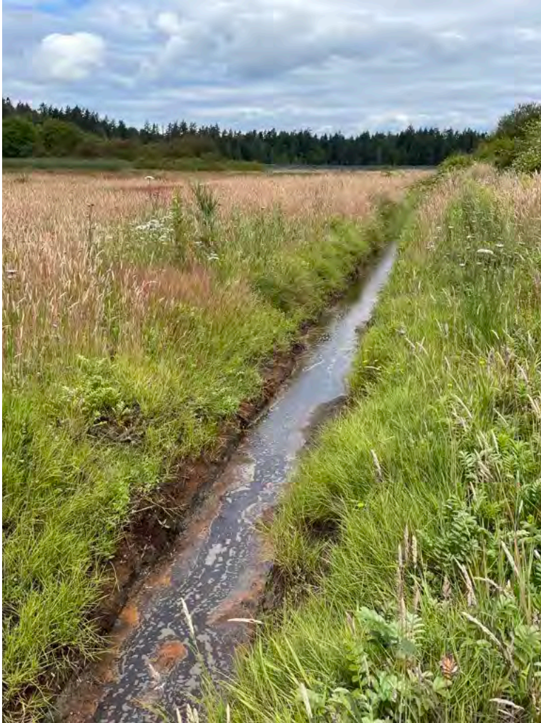
Downstream end of Ditch 2 looking northwest July 16, 2022. The channel is clear. The trail of bubbles were flowing south as expected. Iron bacteria were significantly reduced over last year.
