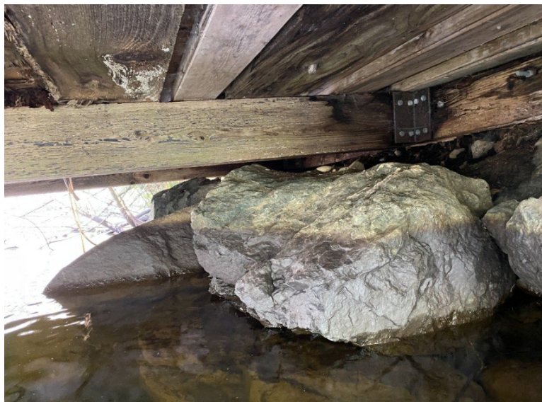
Figure 4: Underside of Deck at Abutment Location.
