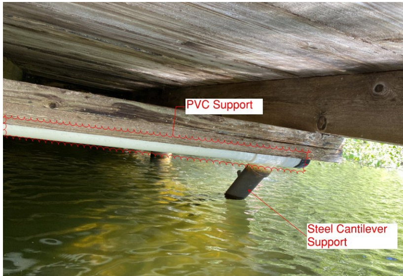
Figure 5: Existing PVC Support Transitioning to Steel Knee Brace.
