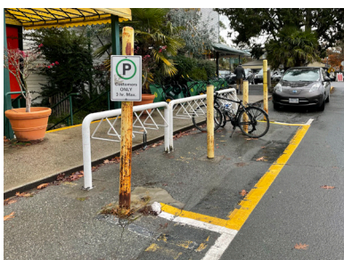
Example of ‘Coat Hanger’ rack type which does not meet best practices
