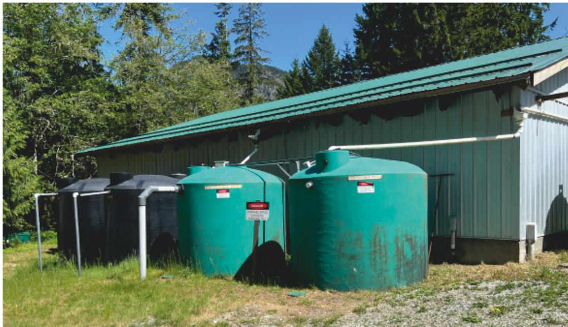
**Figure J. Rainwater Storage Tanks**
