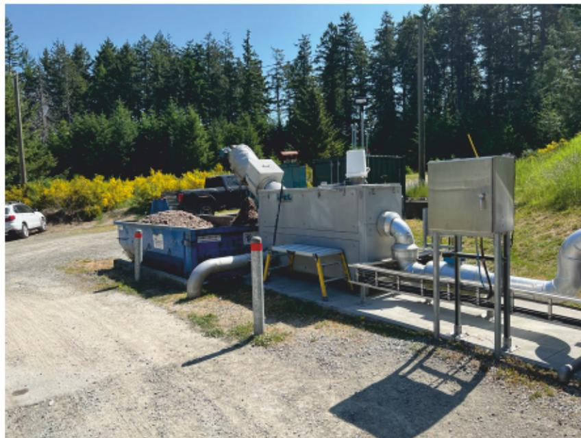
**Figure F. Waste-Stream Receiving Grit Removal and Screening Facility**
