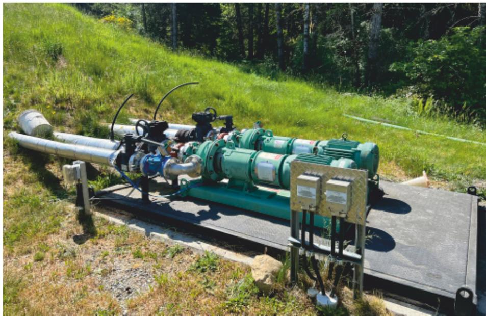
**Figure H. Storage Tank Recirculation Pumps**
