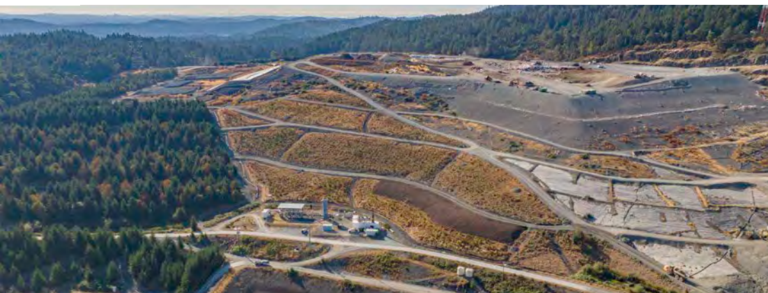
Hartland Landfill and the Landfill Gas Plant
