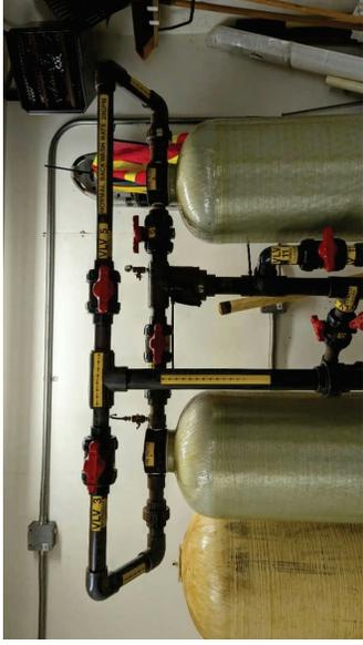
Figure A-14 WTP Arsenic Removal Process
