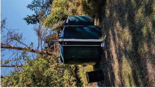
Figure A-6 WTP Backwash Tanks
