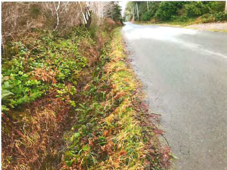
Photo 14. Ditch C flows west along the north side of Invermuir Road.
