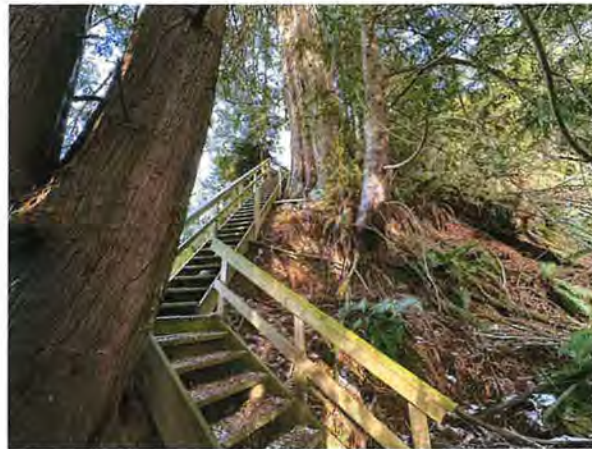
Photo 8. Existing stairs leading to shoreline area.
