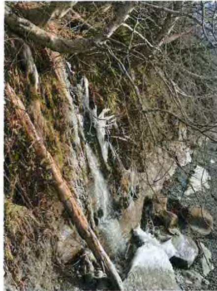
Photo 10. Downstream extent of western-most stream, discharging to the marine environment. January 16, 2024.
