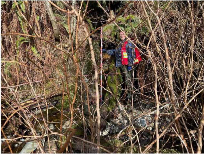
Photo 21: Two meter high vertical barrier to fish passage at the cobble beach interface.
