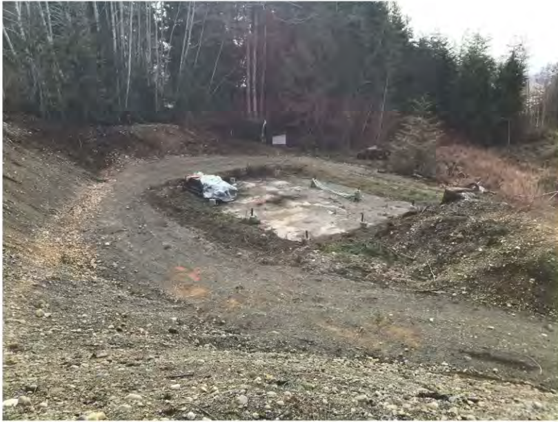
Photo 17: Gravel area with concrete pad.
