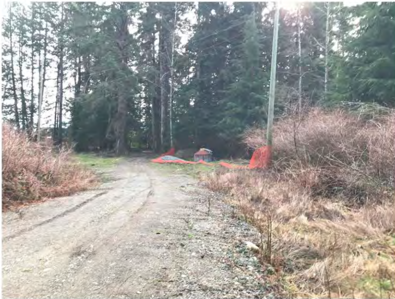
Photo 3. Existing driveway at west of 9333 Invermuir Road with well installed in 2023, proposed pumphouse to be constructed.
