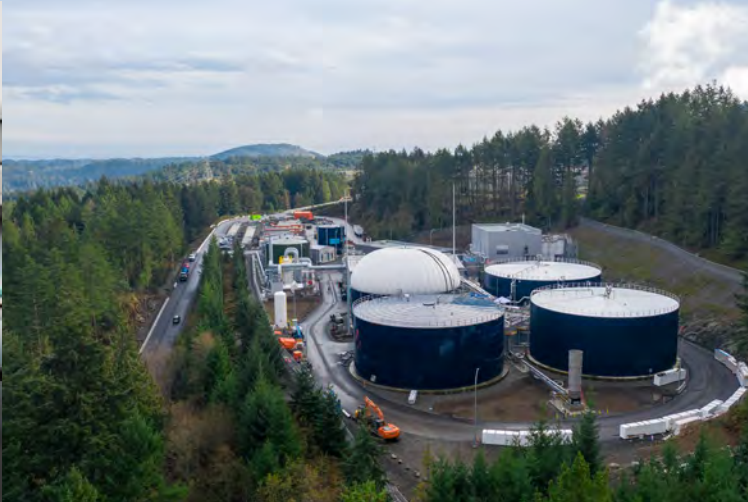
Residual Treatment Facility
