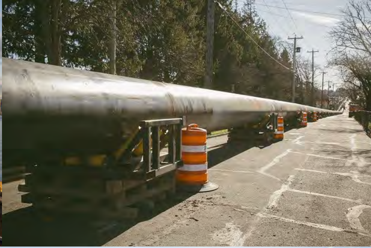
92 km Conveyance System
