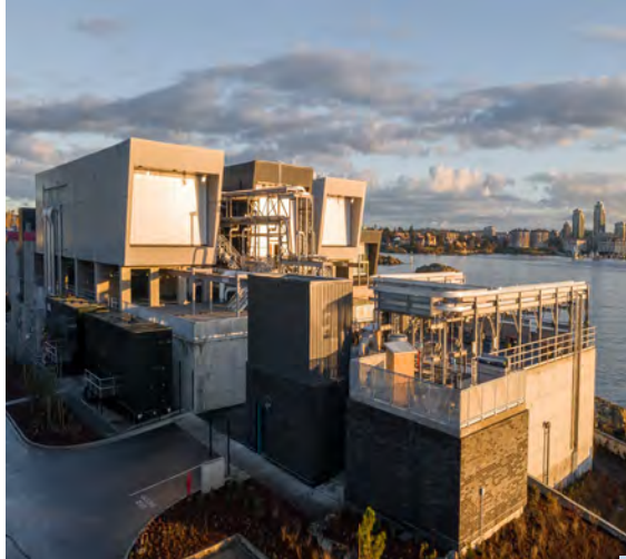
McLoughlin Treatment Plant
