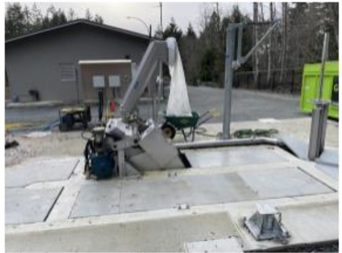
Fine Screen and Washer/Compactor
