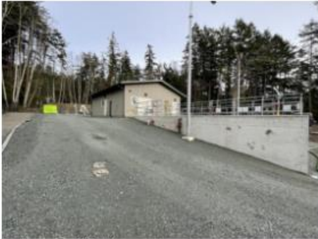
Schooner WWTP and Tanks
