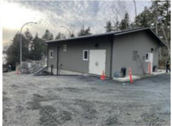
Schooner WWTP Operations Building
