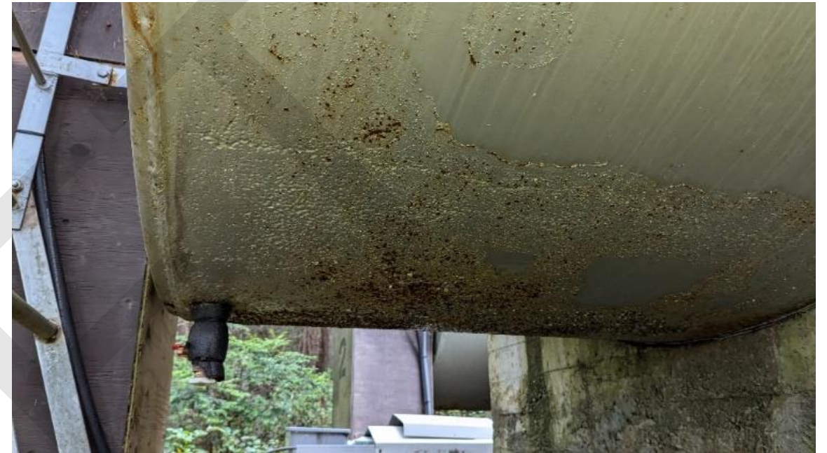
Figure B-4 Flange Connection/Corrosion
