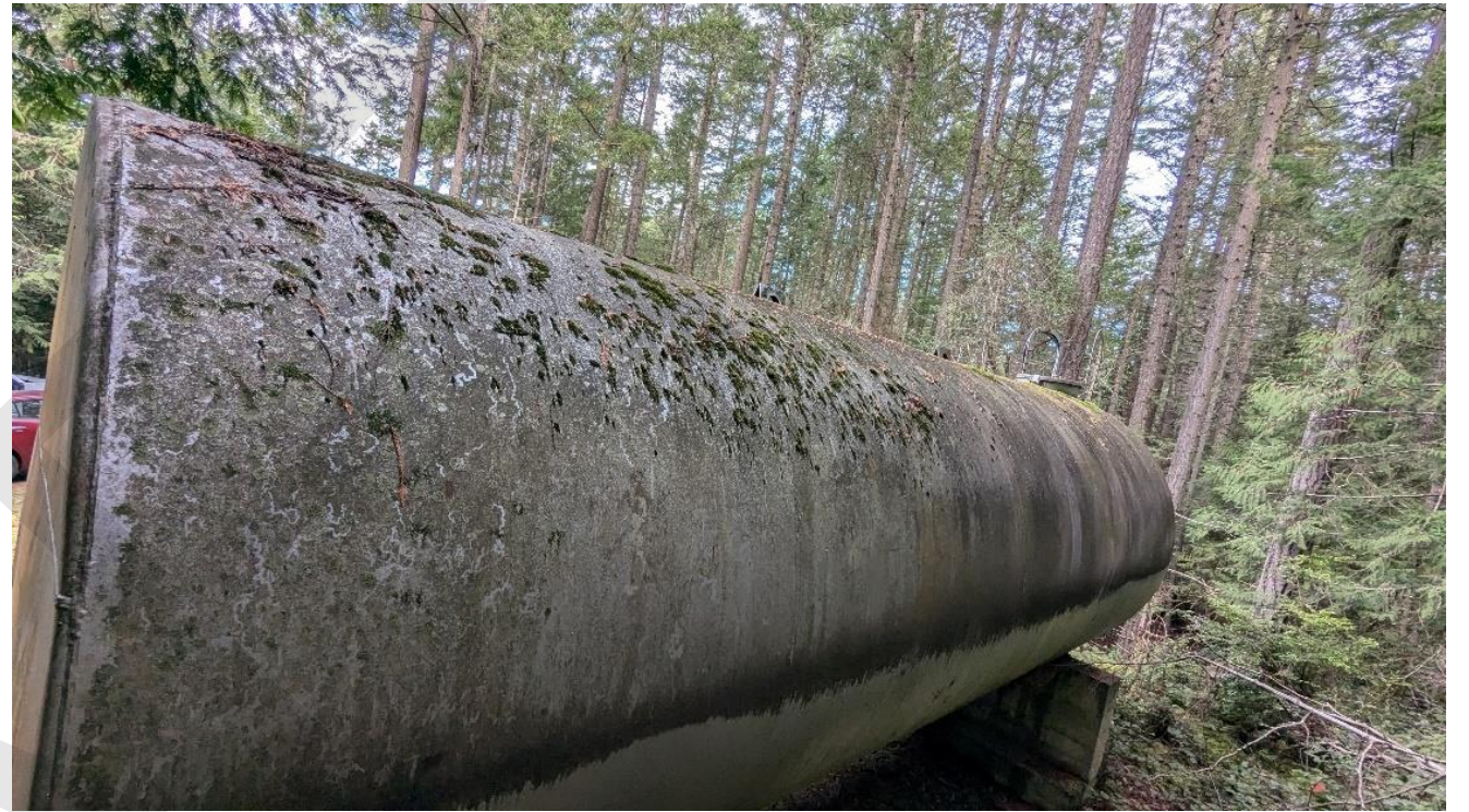
Figure B-6 Exterior Top of Tank
