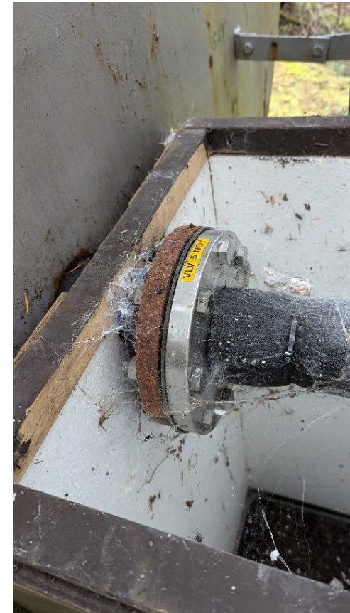
Figure B-4 Flange Connection/Corrosion
