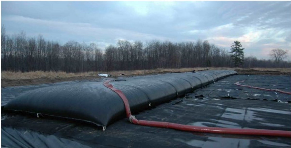
Photos of Geotubes in Operation
