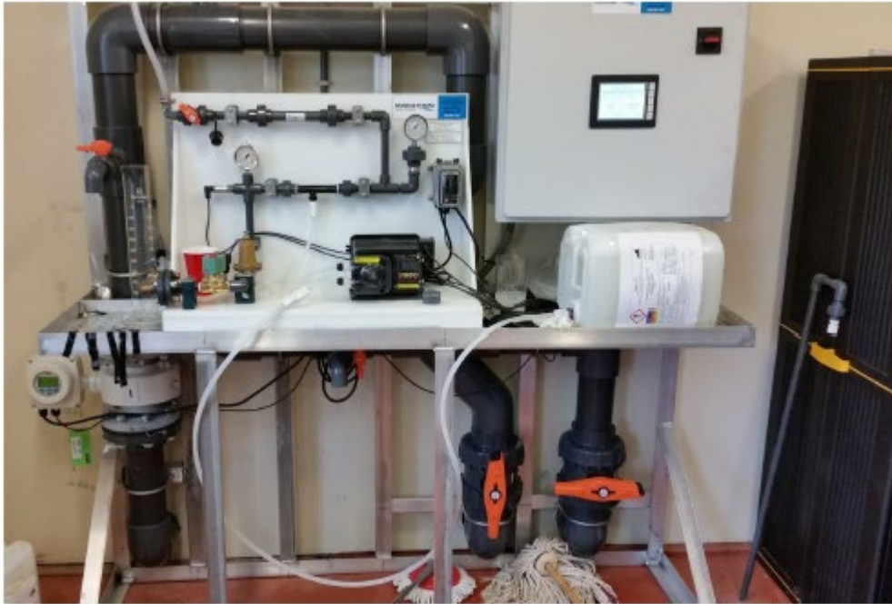
Photos of Equipment Required to Add Flocculant Prior to Entering Geotubes
