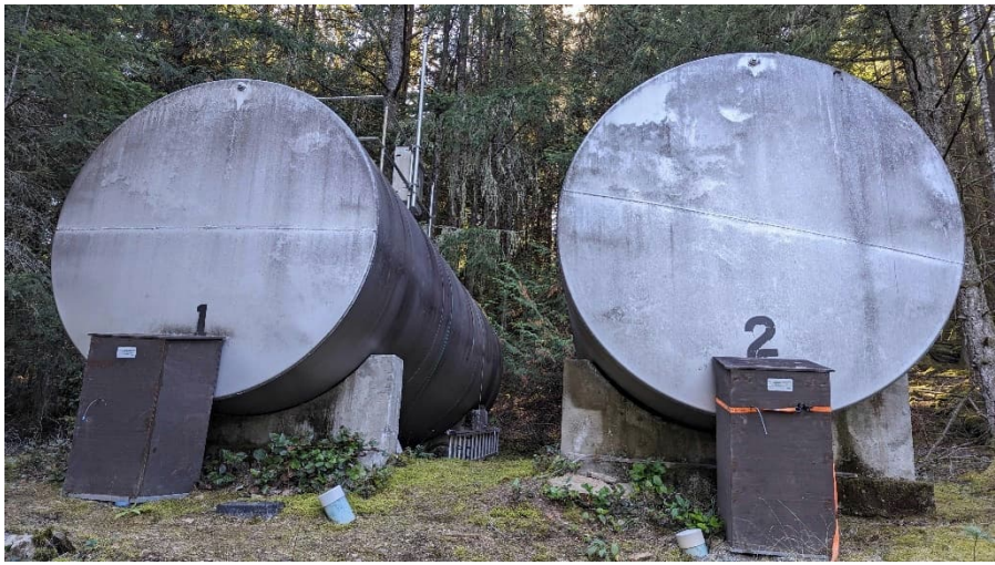
Figure A-13 Existing Reservoir Concrete Saddles
