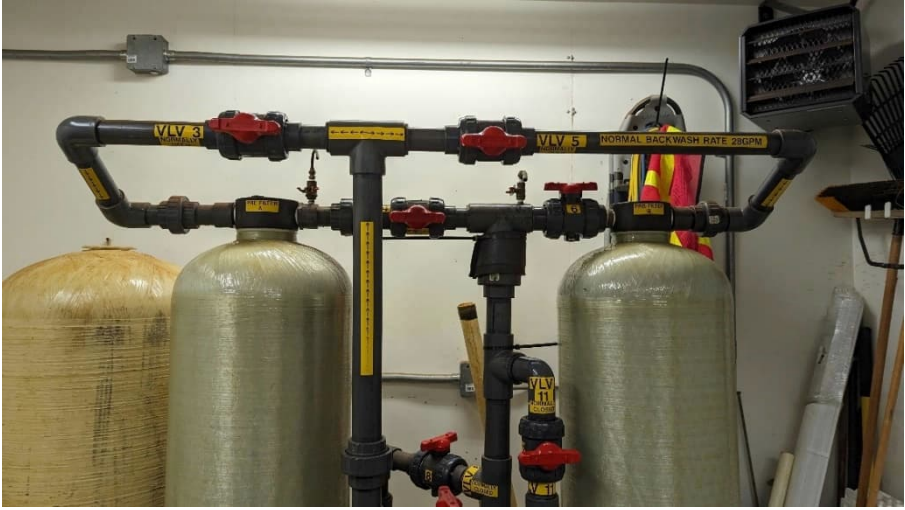
Figure A-14 WTP Arsenic Removal Process
