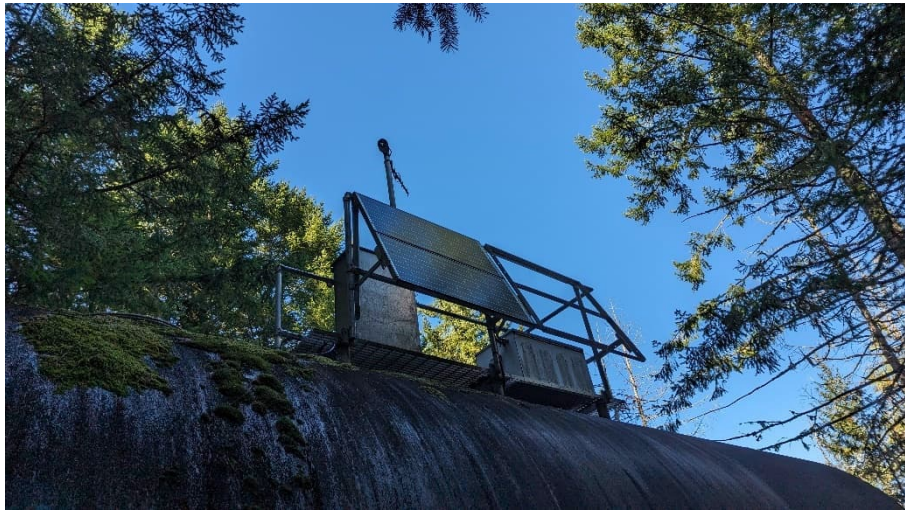
Figure A-12 Existing Reservoir Antenna/Transmitter
