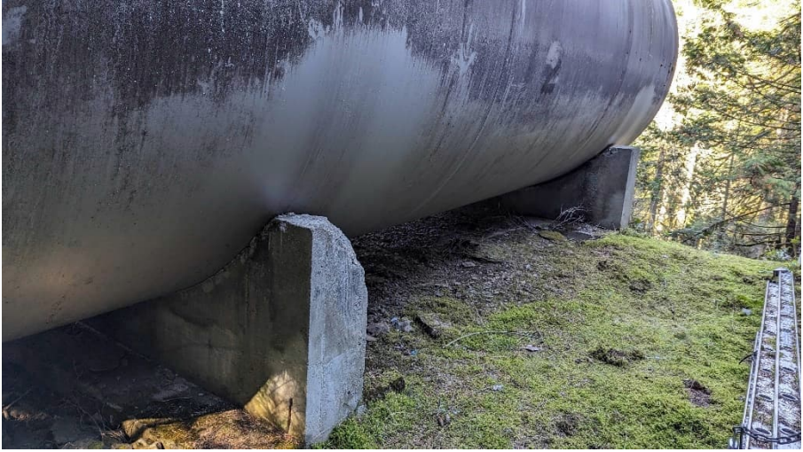
Figure A-13 Existing Reservoir Concrete Saddles
