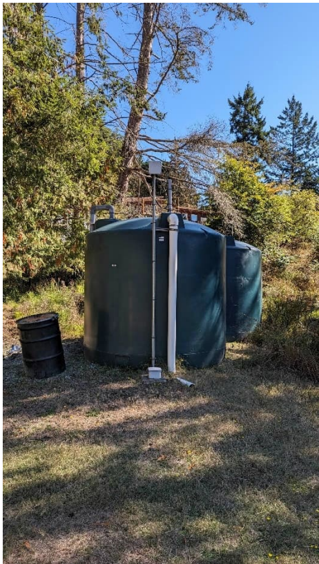
Figure A-6 WTP Backwash Tanks
