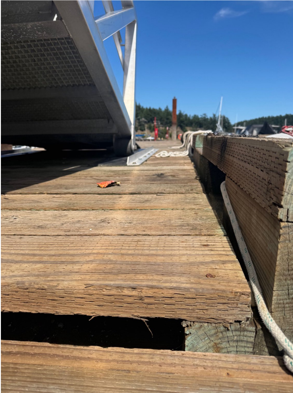
Horizontal gap beneath planks for conduit access
