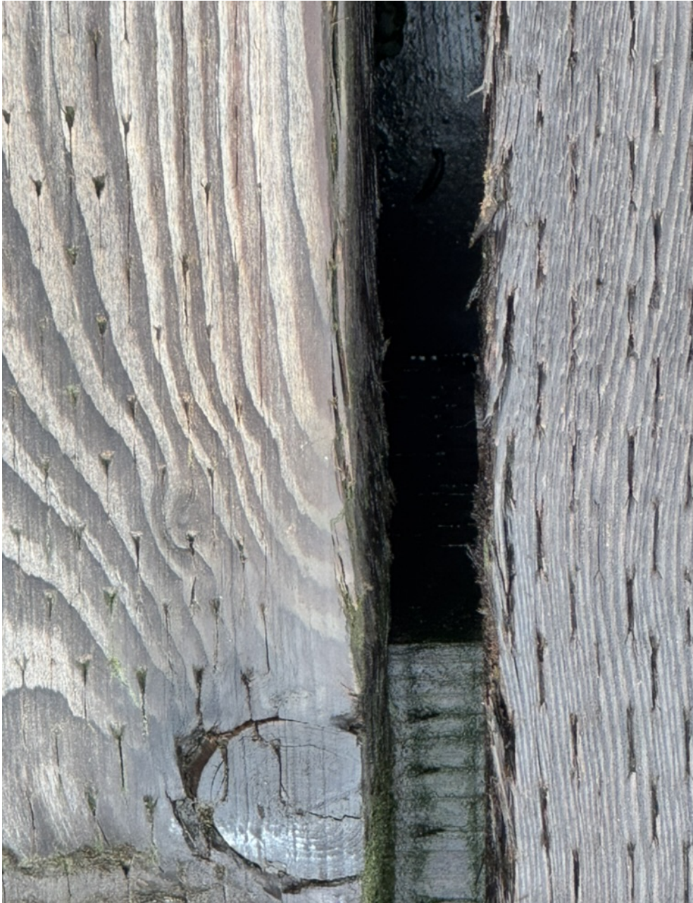
Drop strapping between dock planks
