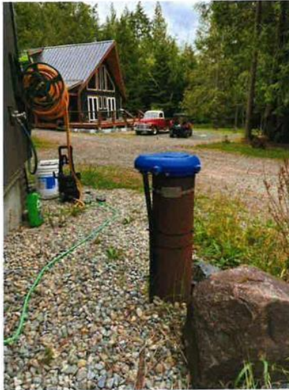
Photo 1. Existing Supply Well WTN 96137
