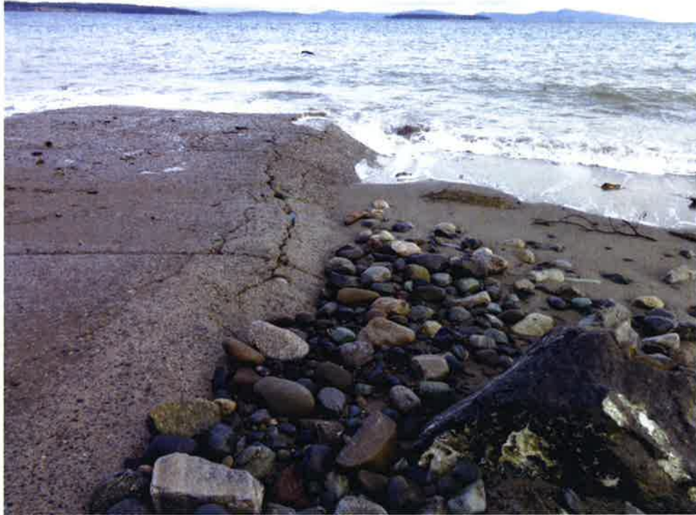
Photograph 6: The southern side of the boat ramp taken facing east on December 19, 2015
