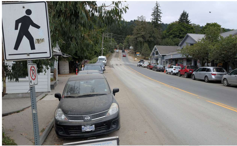
Figure 37: Ganges Alley Crosswalk South Looking West
