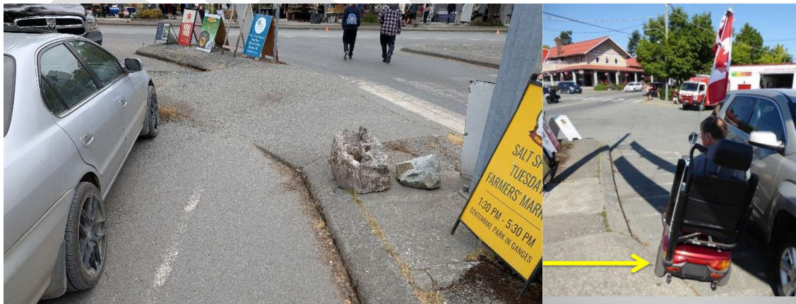
Figure 30: Fulford-Ganges and Lower Ganges Ramp Accessibility (Credit: Gary Lehman)
