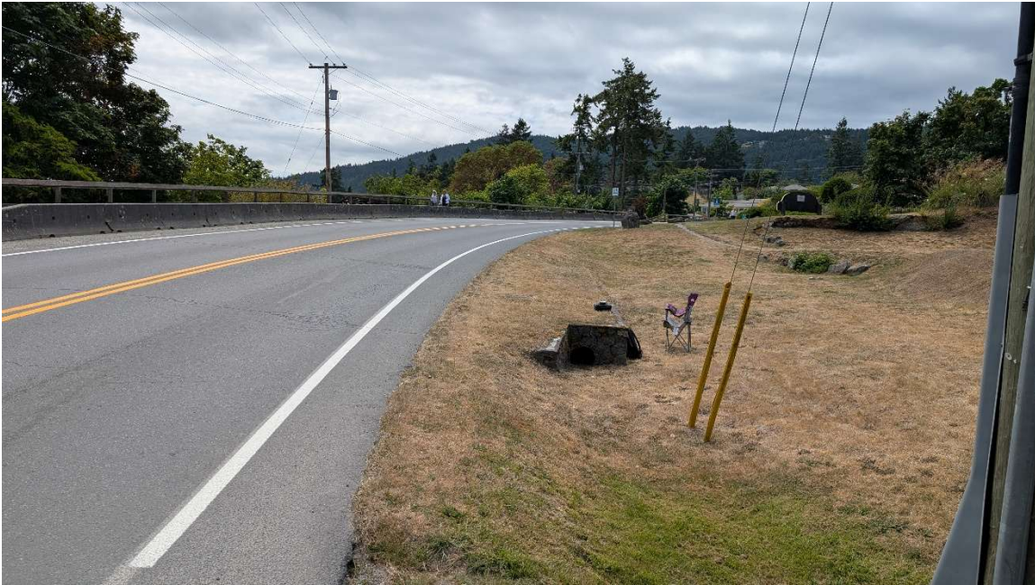
Figure 62: Upper Ganges at Marina West Side Looking South
