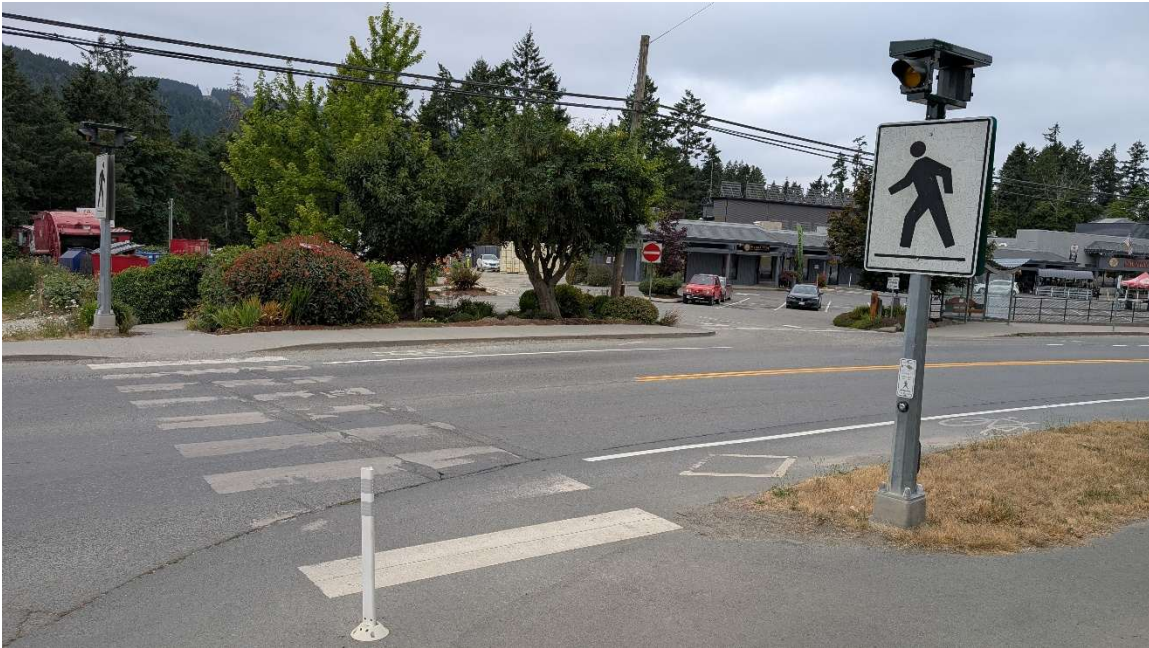
Figure 2: Lower Ganges at Crofton Crosswalk
