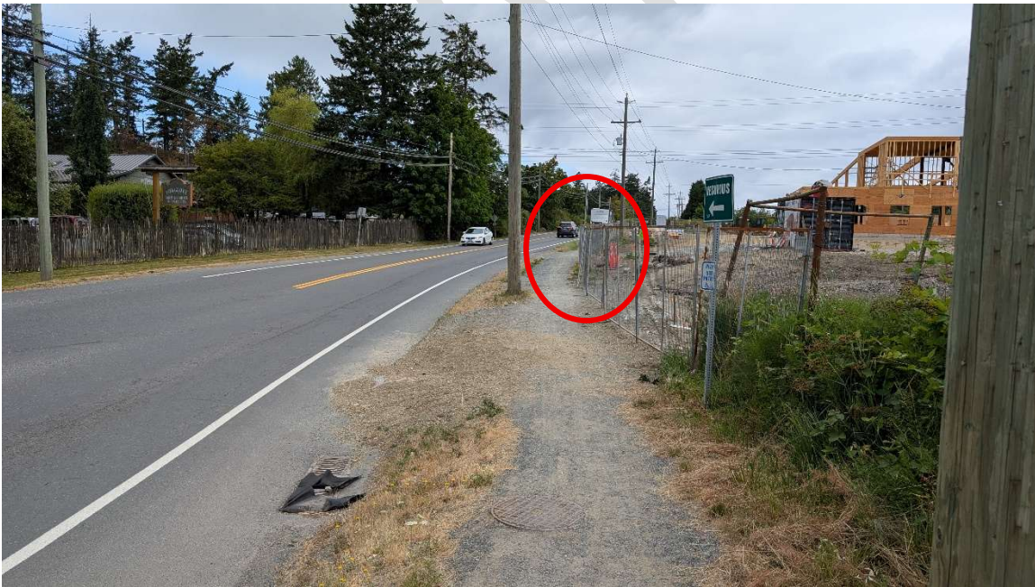
Figure 52: Lower Ganges / Atkins Northeast Corner Looking West
