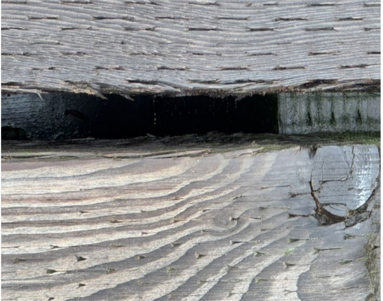
Photograph: View between deck planks. Floatation and beams beneath.
