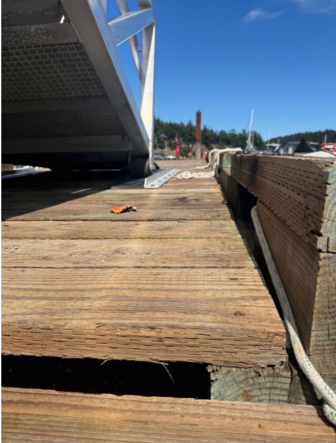
Photograph: end of dock showing structural detail
