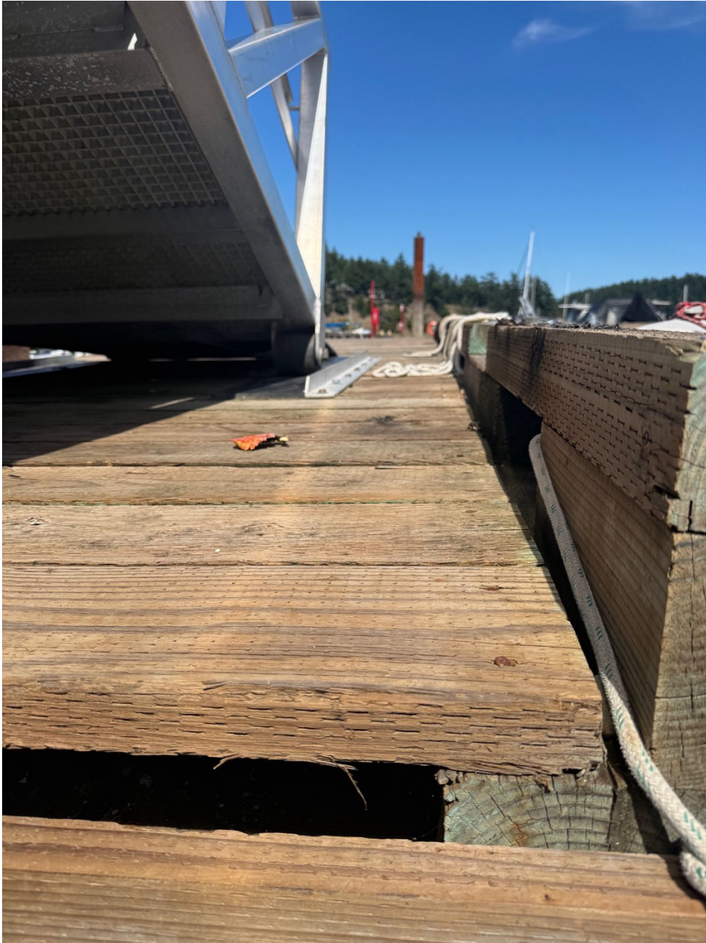
Horizontal gap beneath planks for conduit access
