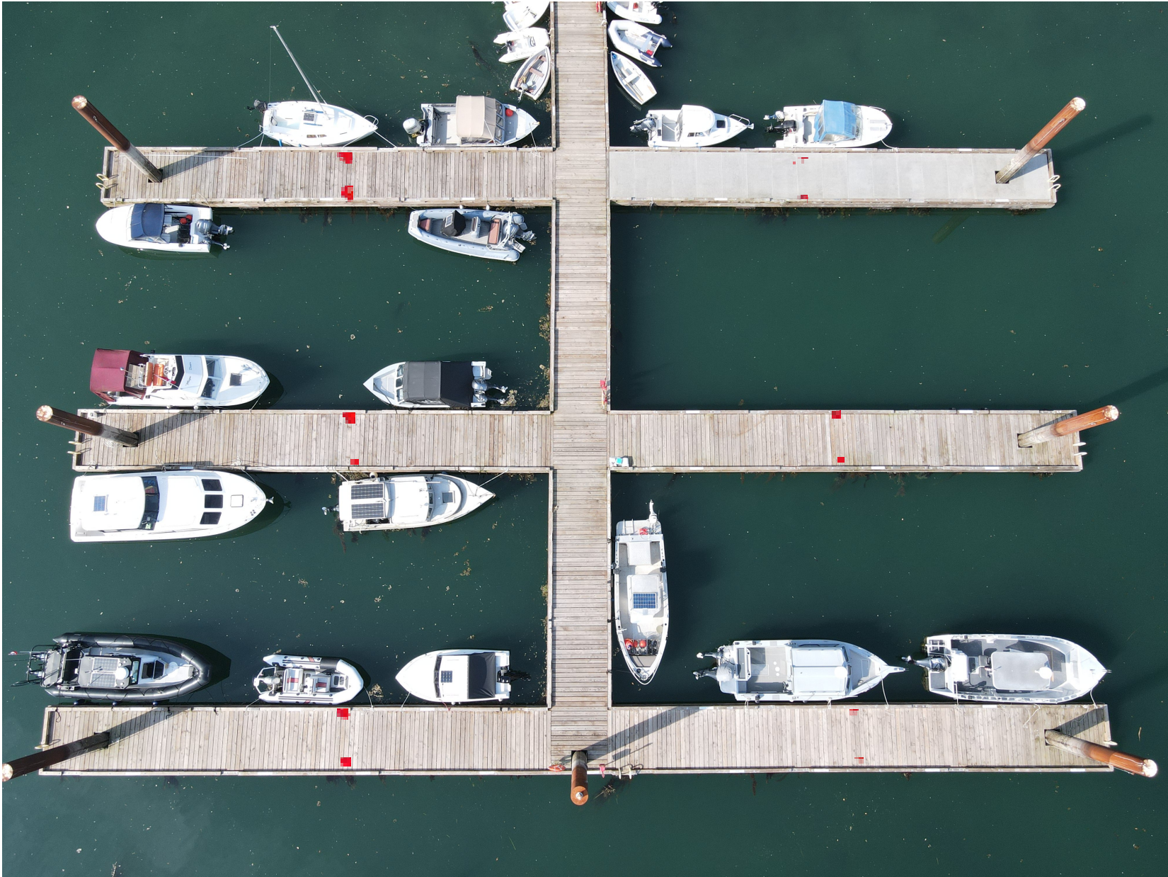
Anson Road Dock. Six fingers. This view depicts the type of boat with summer moorage. ■ = 12 x PEDESTALS LOCATION
