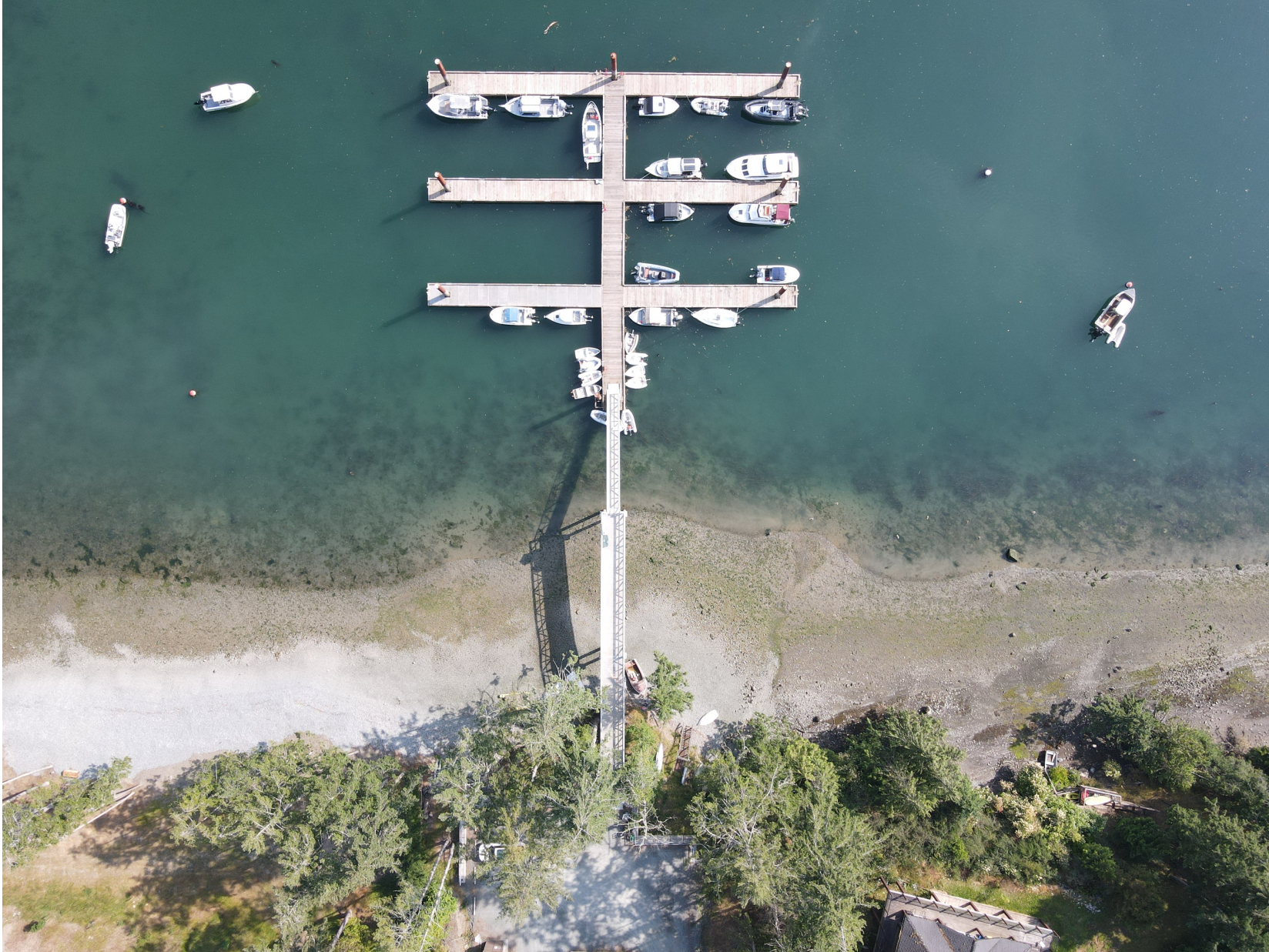
Overview of dock from head of dock along the solid ramp, then hinged ramp, to the 6 fingered dock.
