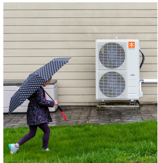
Heat pump outside family home
