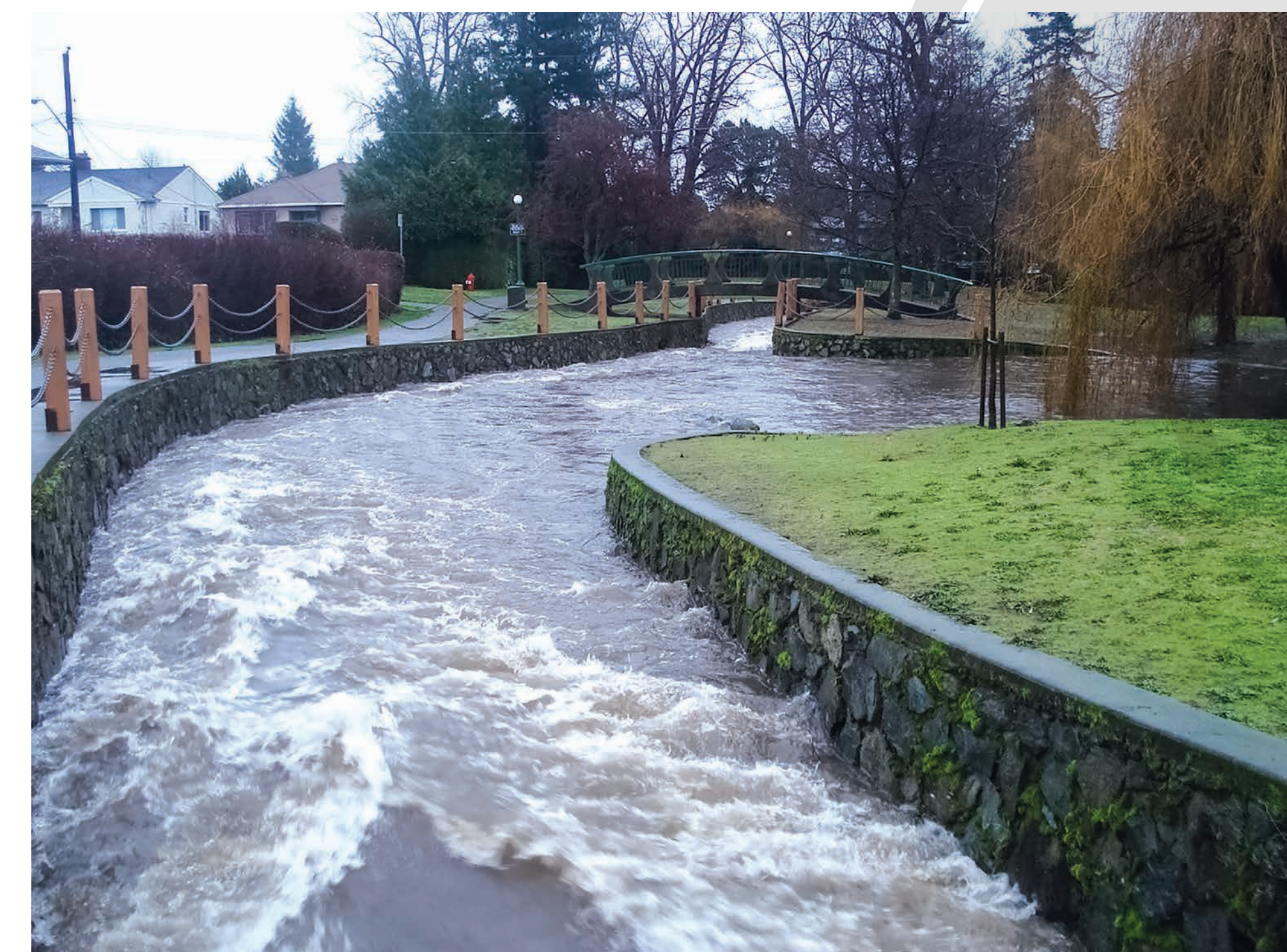
Channelization and piping of the creek has resulted in habitat loss, poor water quality, flooding and erosion. Stormwater flows off impervious surfaces (e.g., roads, roofs) into stormdrains that lead directly to the creek, resulting in fast flows during heavy rain events.
