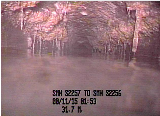
Grease adhering to sewer pipes below Wharf Street.
