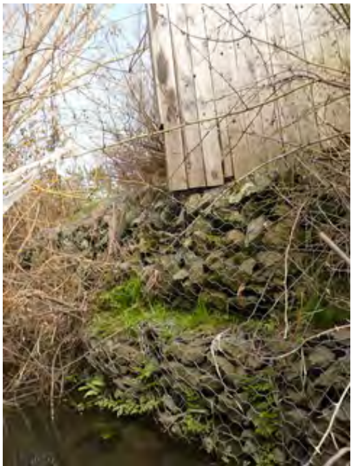
Plate 29: The property at 1875 Haultain comes to a point at the edge of Bowker Creek and is stabilized by gabions.
