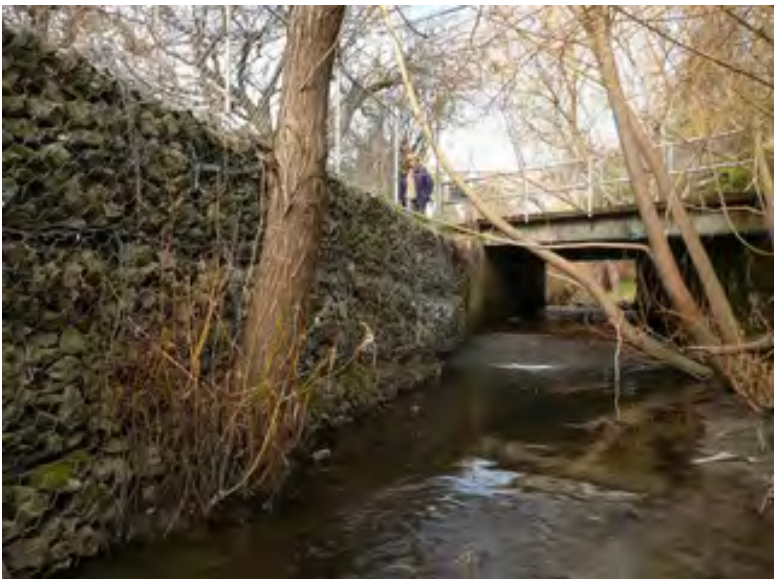
Plate 30: Gabions are controlling erosion at the top end of this reach, allowing for a streamside footpath on the west bank.
