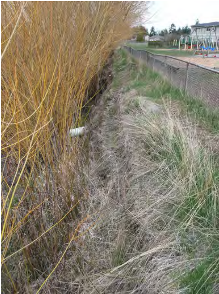
Plate 24: Upstream of the demonstration restoration section showing dead bioengineering along the east bank, behind thriving yellow willow growing on the channel bottom.
