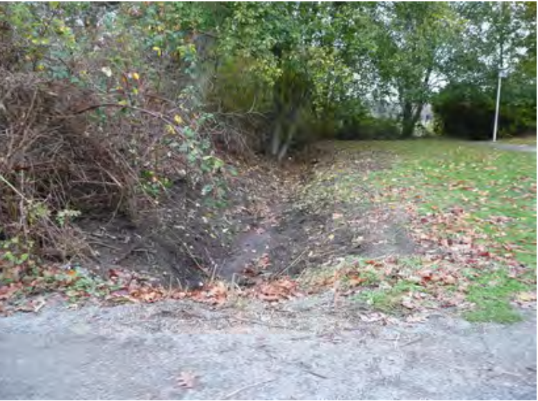
Plate 65: Runoff comes from the Fraser parking lot and is delivered to the channel both overland and through this ditch.
