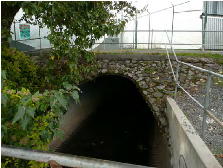
Culvert exiting from under the tennis bubbles at the top of Reach 3
