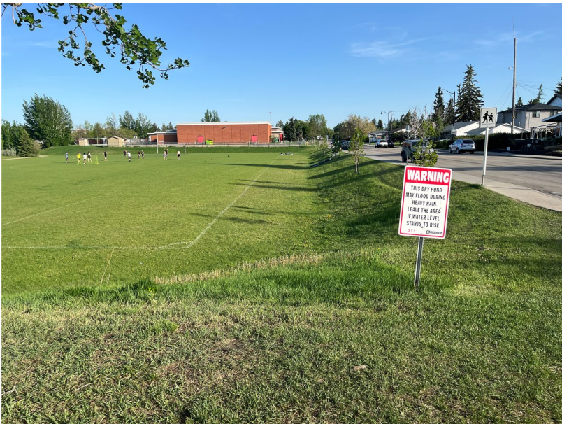
Example of a Dual Use Dry Pond on school playing field in Edmonton AB.
