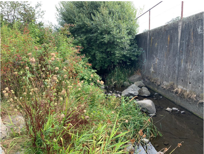
Restored channel and north bank at Oak Bay High School. Primarily native vegetation with some reed canary grass along the channel. Constructed willow bench against south wall adjacent to the running track.
