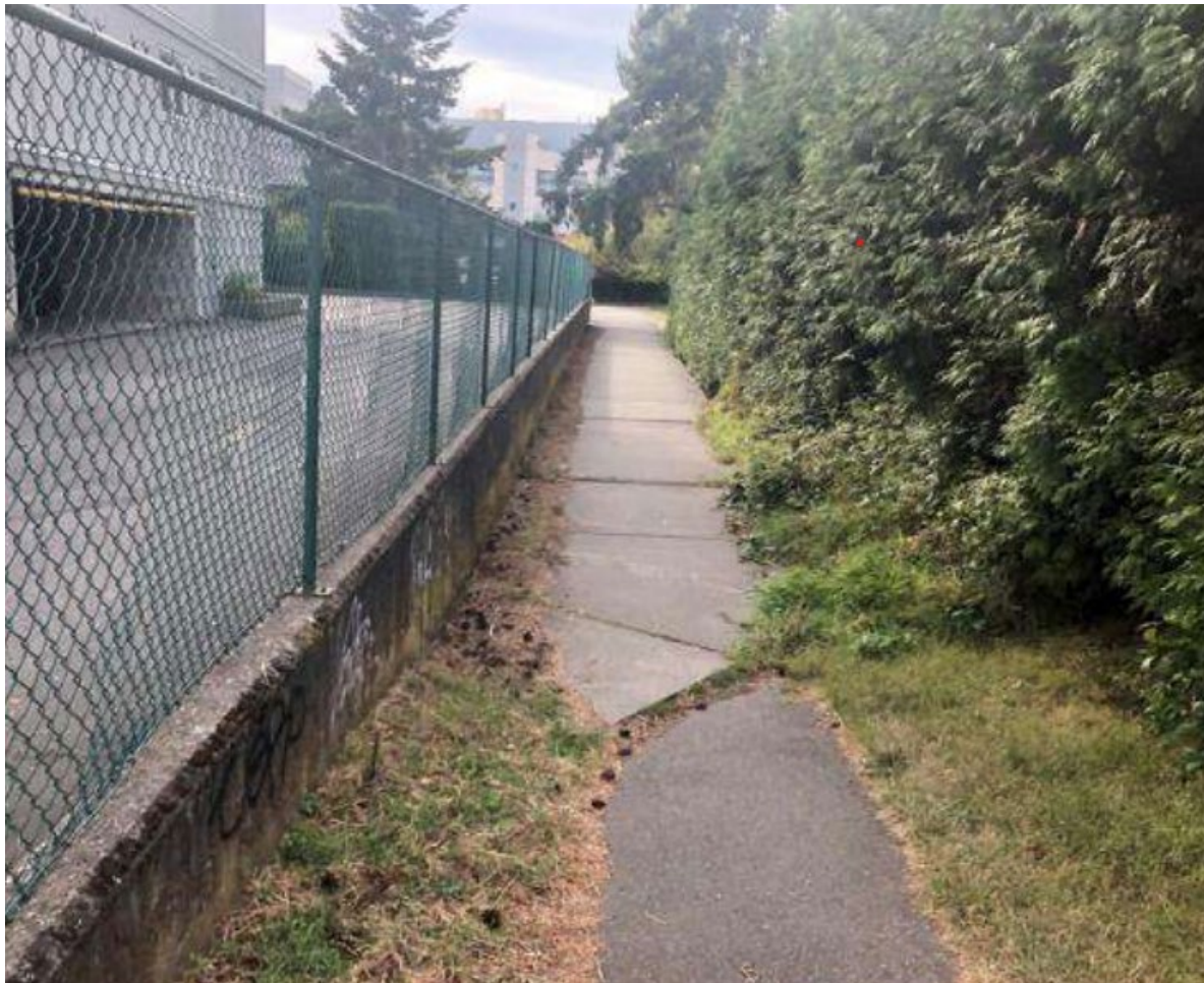
Existing walkway west of Foul Bay Road along Bowker Creek piped section.
