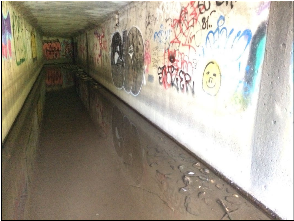
View into culvert from Reach 7 at Richmond Road
