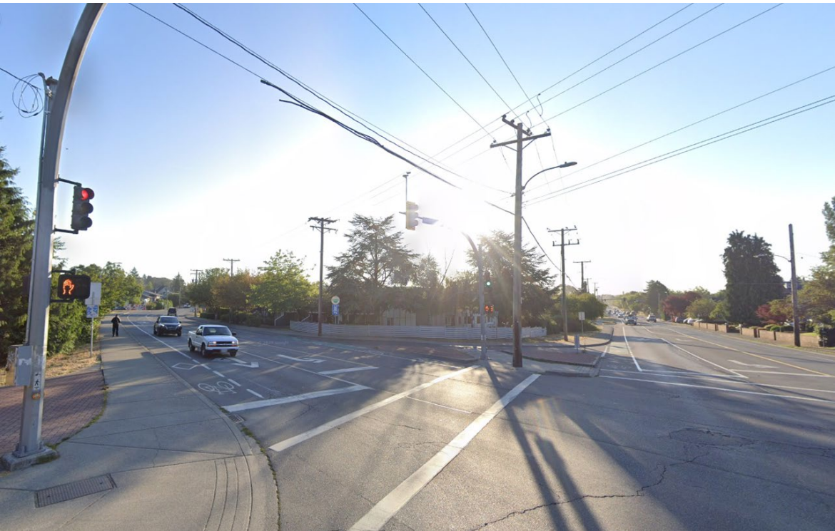
Start of underground section of Bowker Creek at corner of Cedar Hill Road and North Dairy Road.
