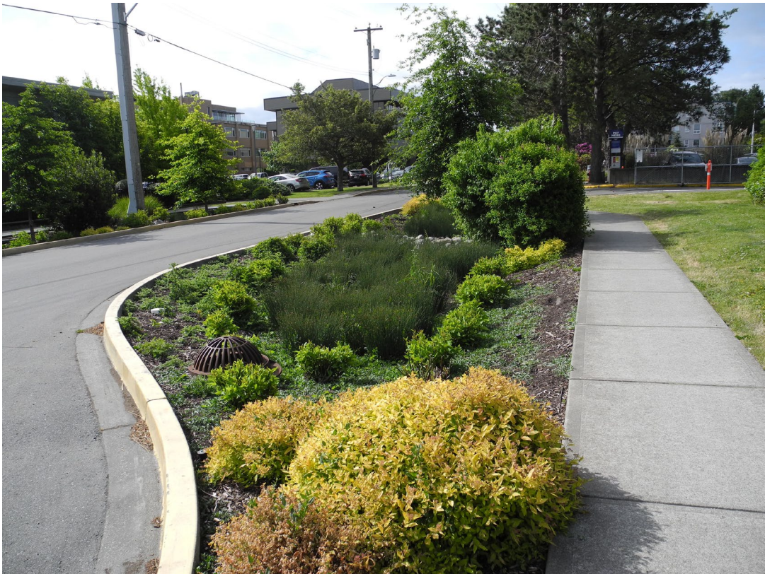
Photo 3. Trent Street Rain Garden, City of Victoria
