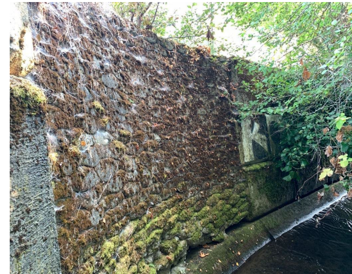
1564 North Dairy Road concrete sandbags.
