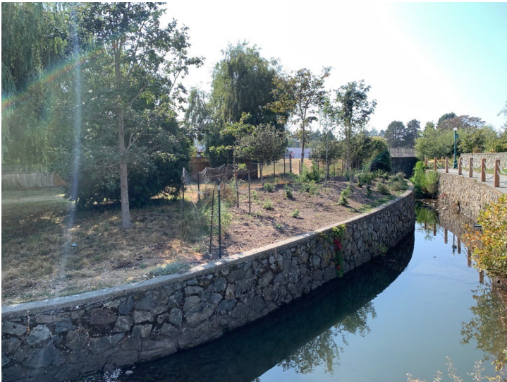
Concrete channel and new riparian plantings by the District of Oak Bay and Friends of Bowker Creek Society.
