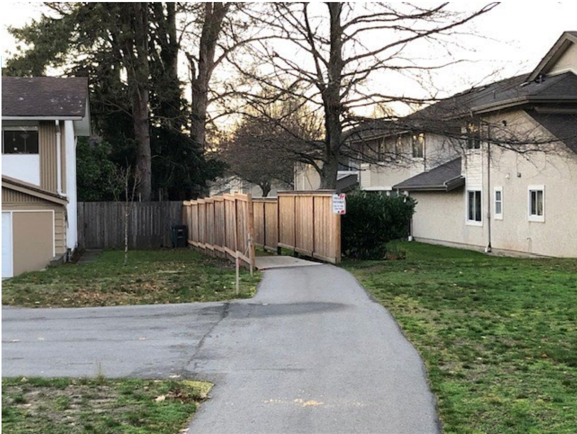
Beginning of culverted section near UVic on Gordon Head Road
