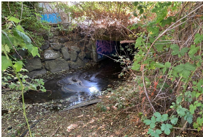
Riprap on west bank at the Pearl Street culvert.
