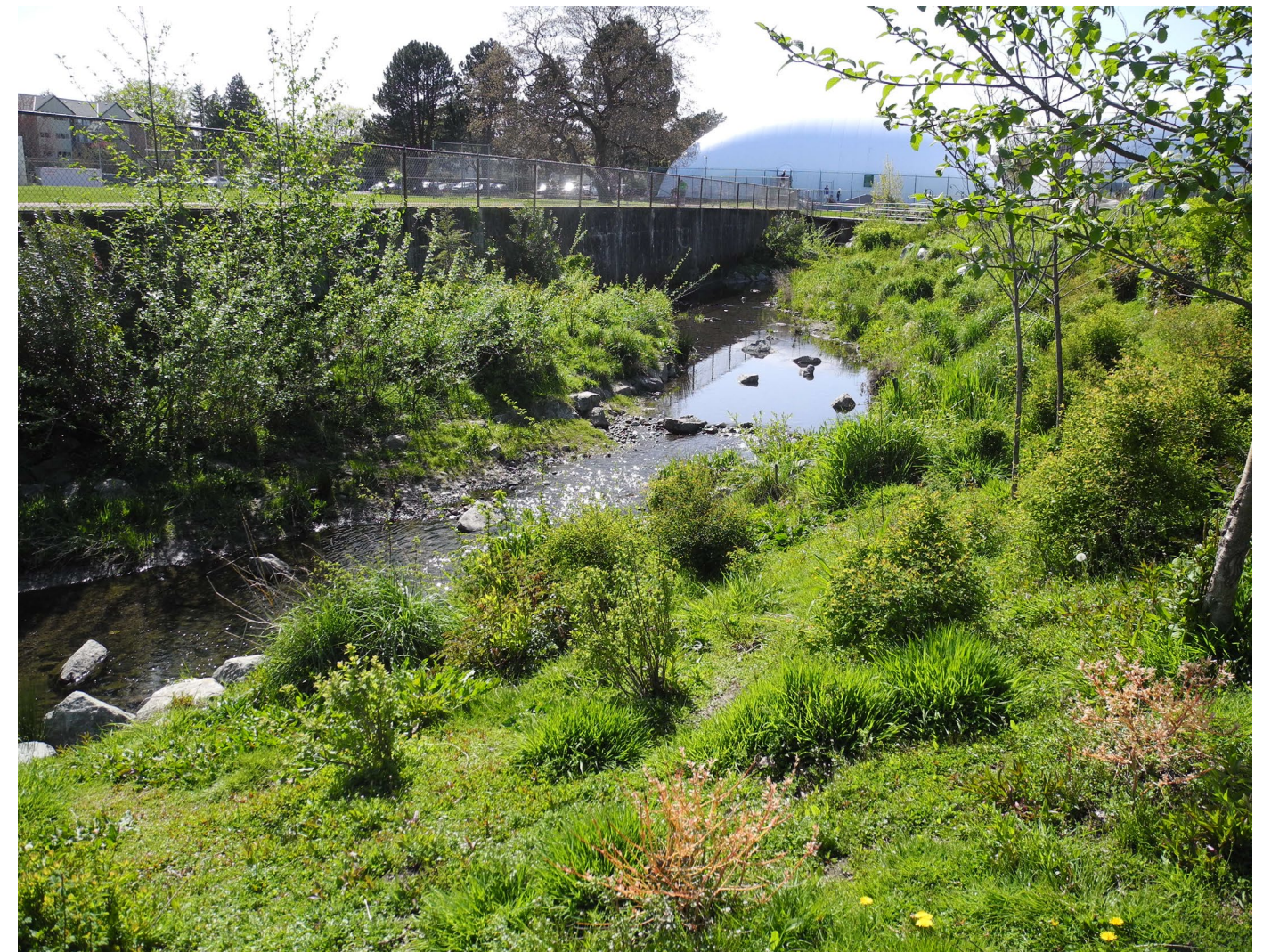
Photo 1. Completed Bowker Creek Restoration at Oak Bay High School
