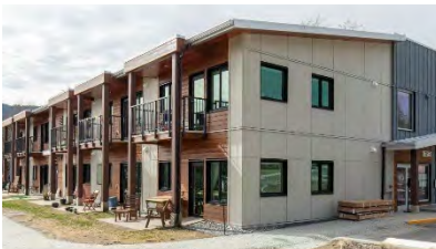
132 Corbett Rd. Phase II Opened 2020
