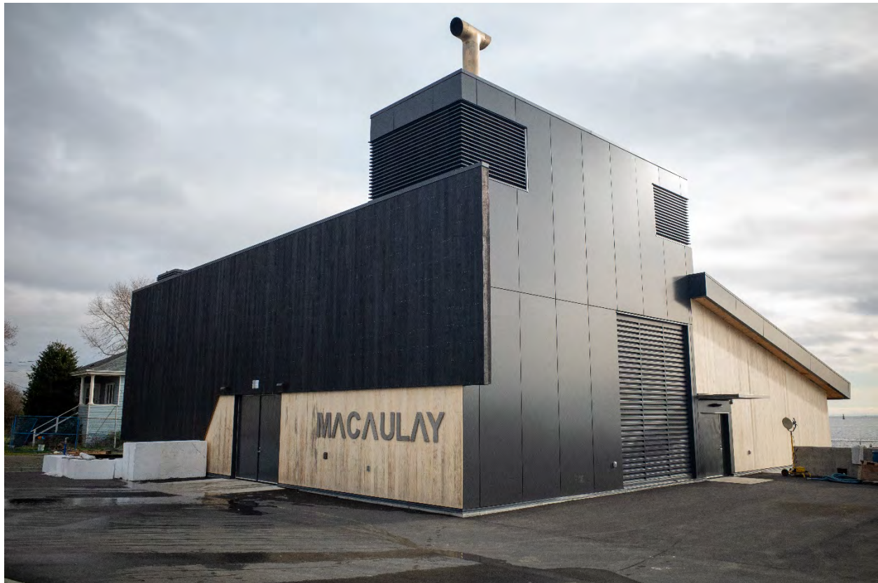
Figure 9 – Macaulay Point Pump Station
