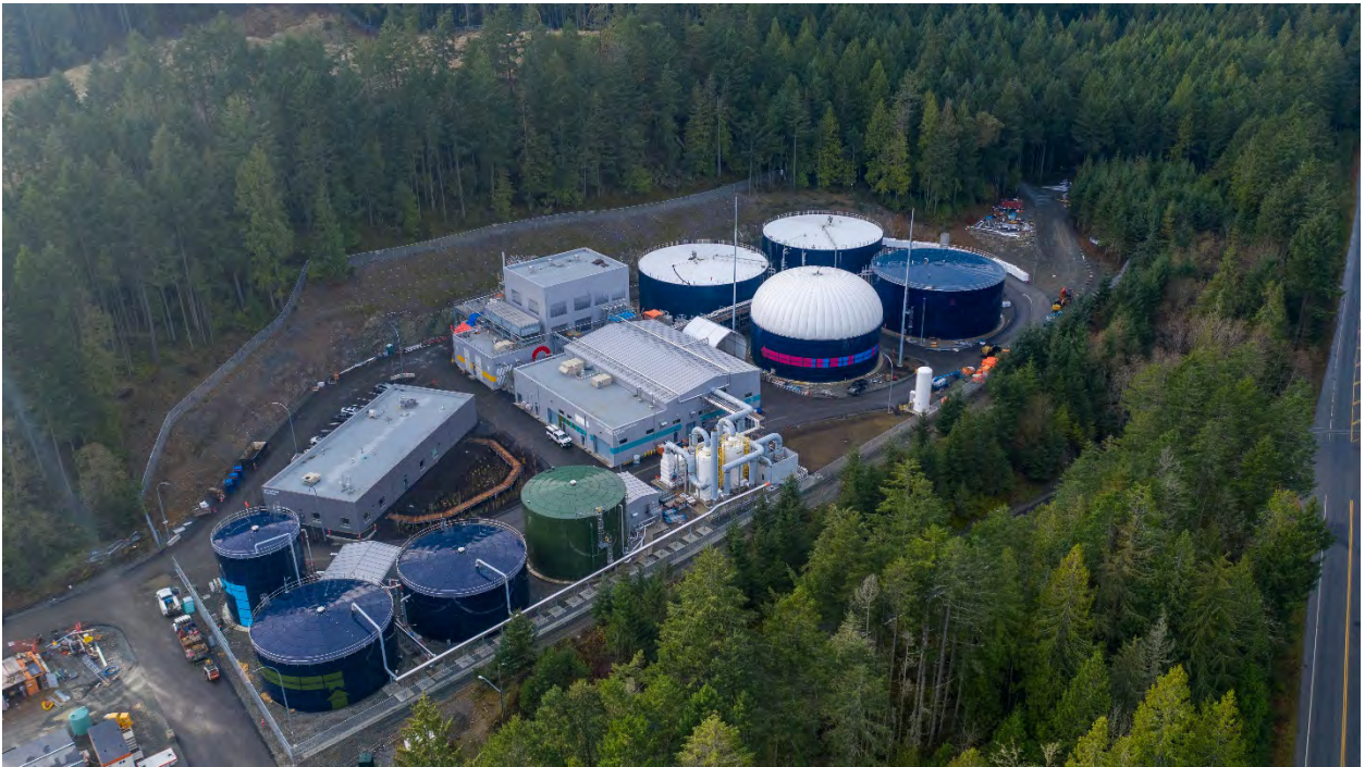
Figure 3 – Looking southwest toward the Residuals Treatment Facility
