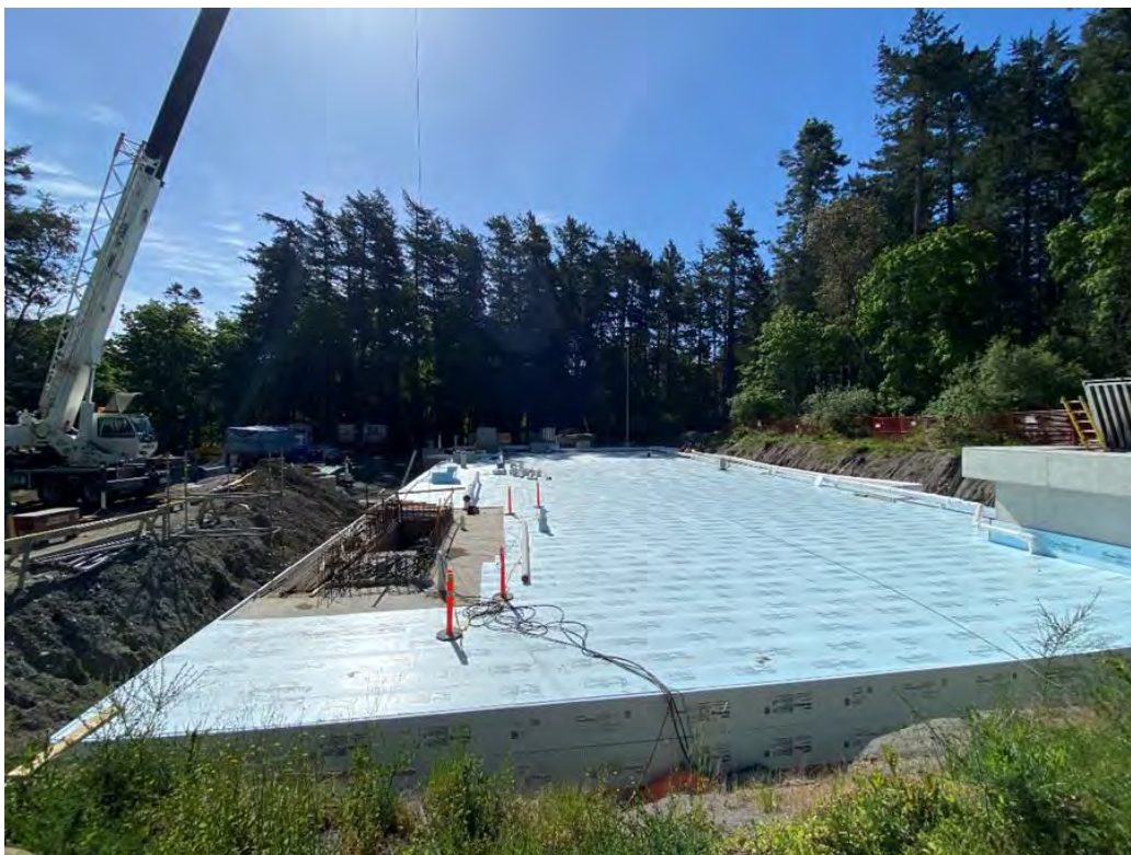
Figure 14 – Arbutus Attenuation Tank (Construction in progress)
