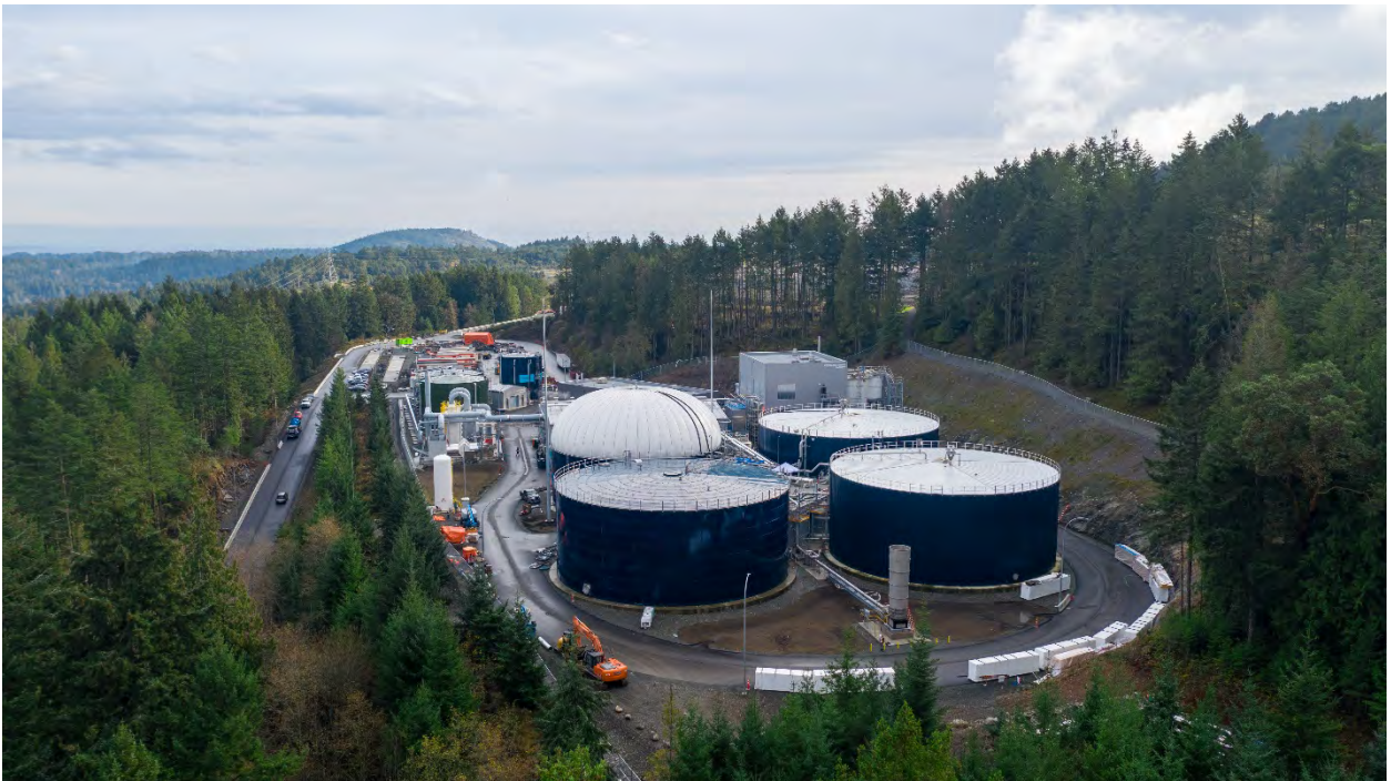
Figure 4 – Looking east toward the Residuals Treatment Facility
