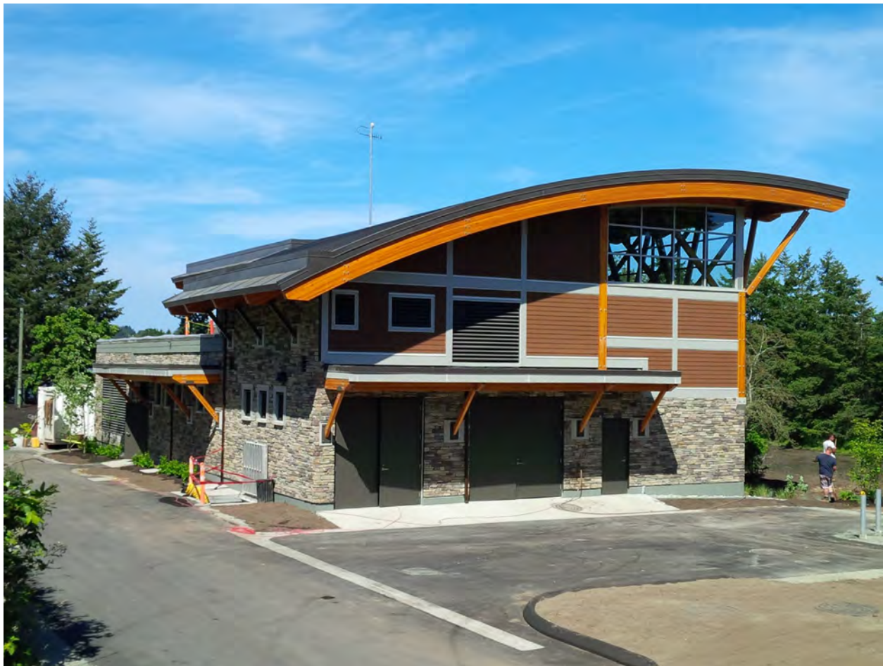
Figure 11 – Craigflower Pump Station
