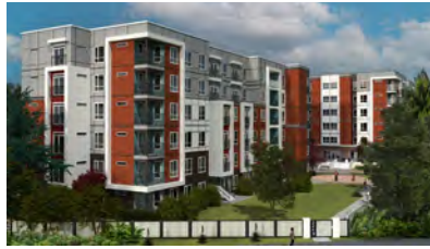
RHFP/BC Builds - Campus View 2027
