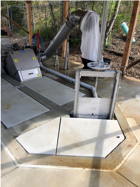
Screen and Discharge Chute
