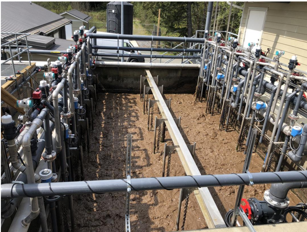
Membrane Bio-reactor Tank
