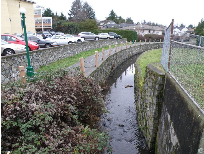
Oak Bay High on left, municipal recreation centre on right, creek at typical flow. NOTE: new school will be relocated on site well away from creek & current buildings demolished.
