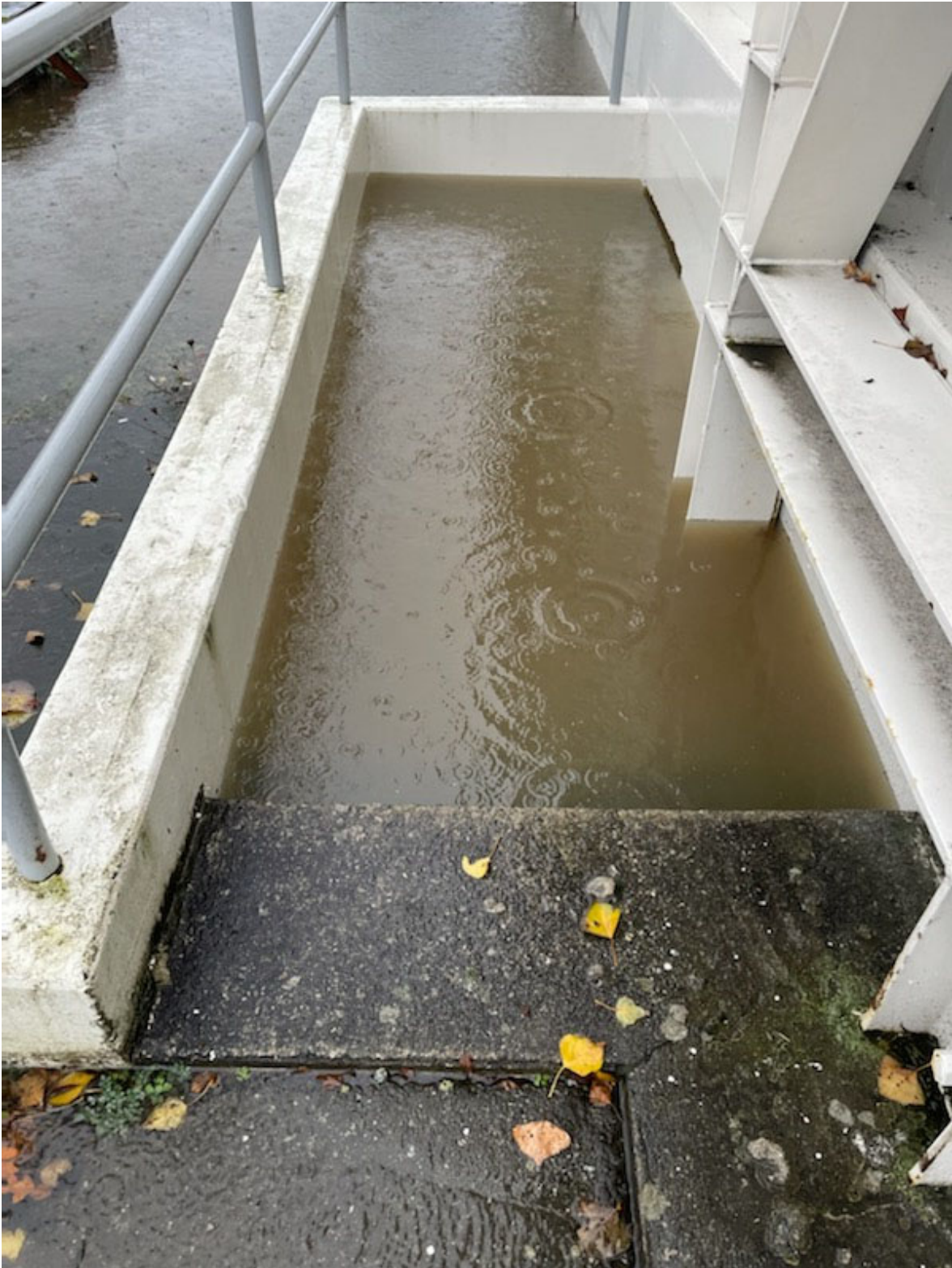
Photo of max wastewater level in Sidney pump station wet well staircase on Nov 15, 2021
