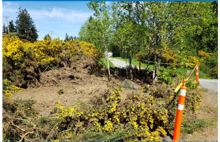
Removing Gorse along the Galloping Goose Regional Trail
